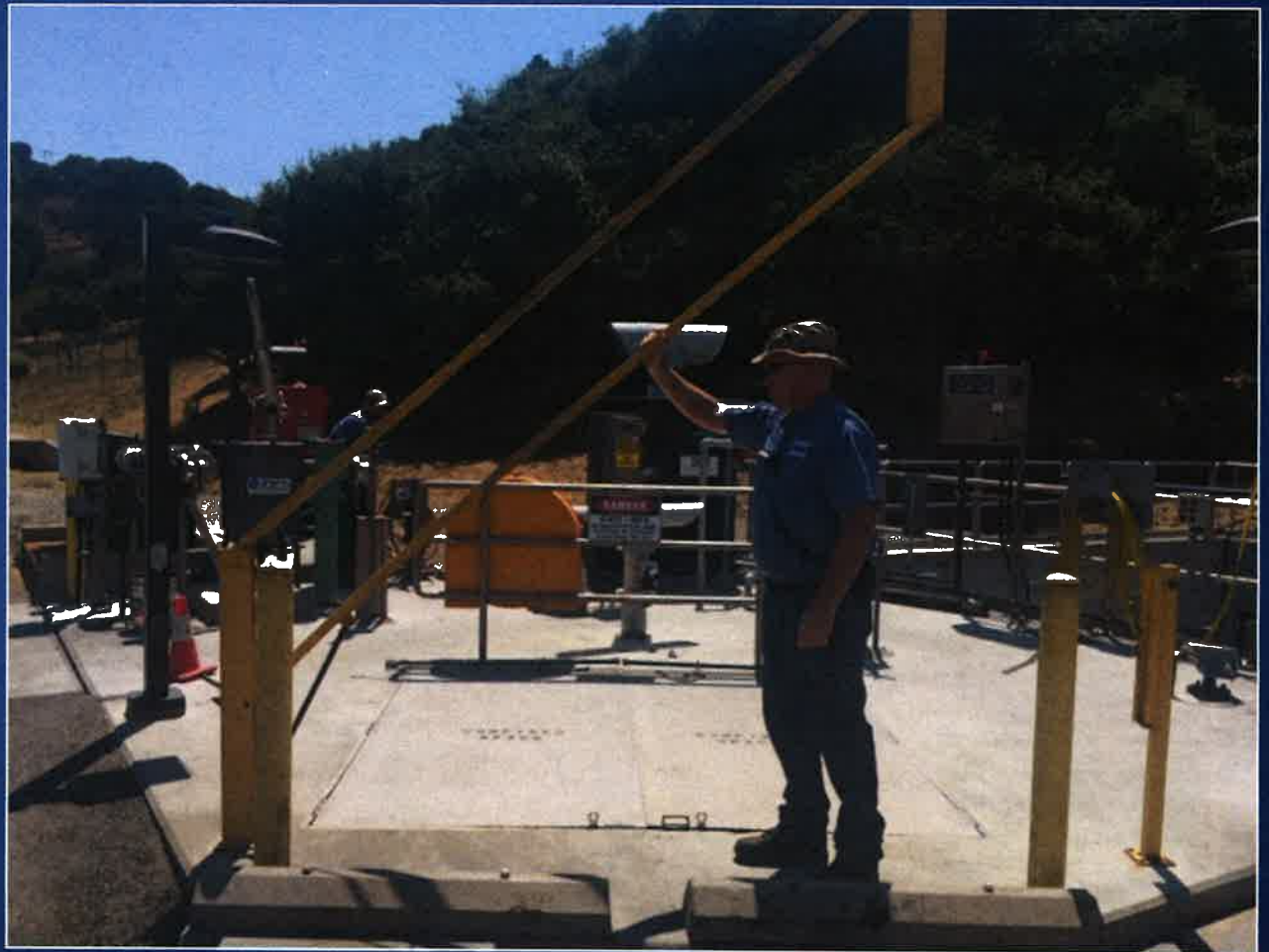
Operator demonstrating Safe Access Gates
