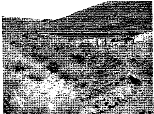
Photograph 6. – View of the last sump in the series (Sump 27). Breckenridge road in the background.
