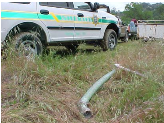
Photo 9. Various aboveground flexible hoses adjacent to septic discharge areas
