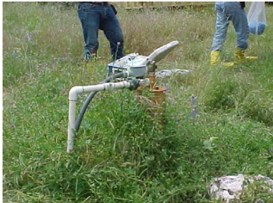
Photo 13. Owens' domestic well adjacent to a septic discharge area and flexible hose
