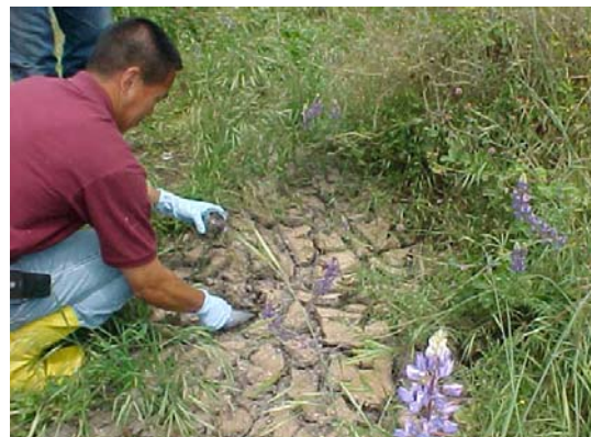
Photo 12. Location of soil sample 3 (note evidence of septic discharge between well and 3-inch flexible hose)
