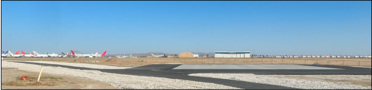
Photo 5.2: A portion of the airfield of Former George AFB, currently Southern California Logistics Airport.
