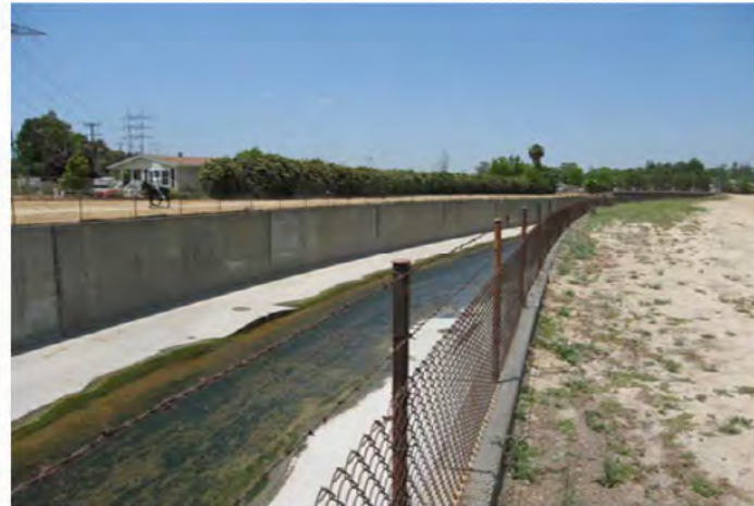
Burbank Western Channel
