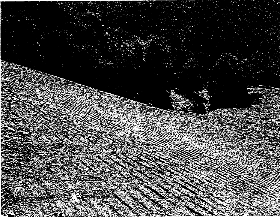
9/25/2009 Site 8 reconstructed by filling in slide body and sloping to a 2:1 slope
