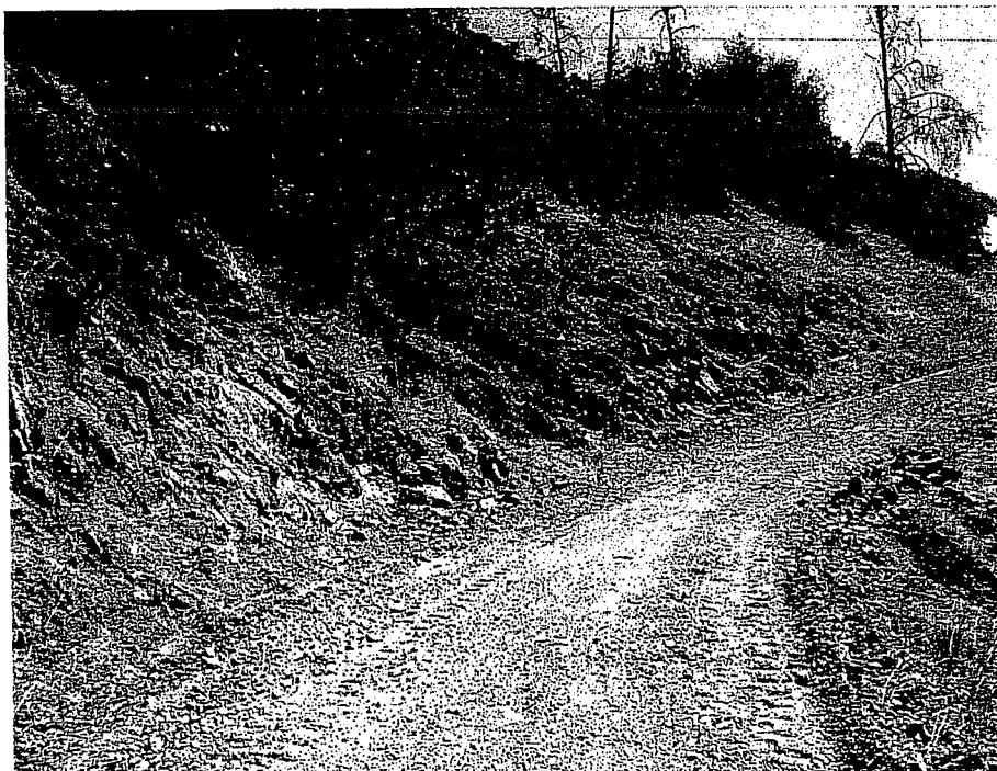
9/25/2009 new road fill across ephemeral swale with no drainage structure
