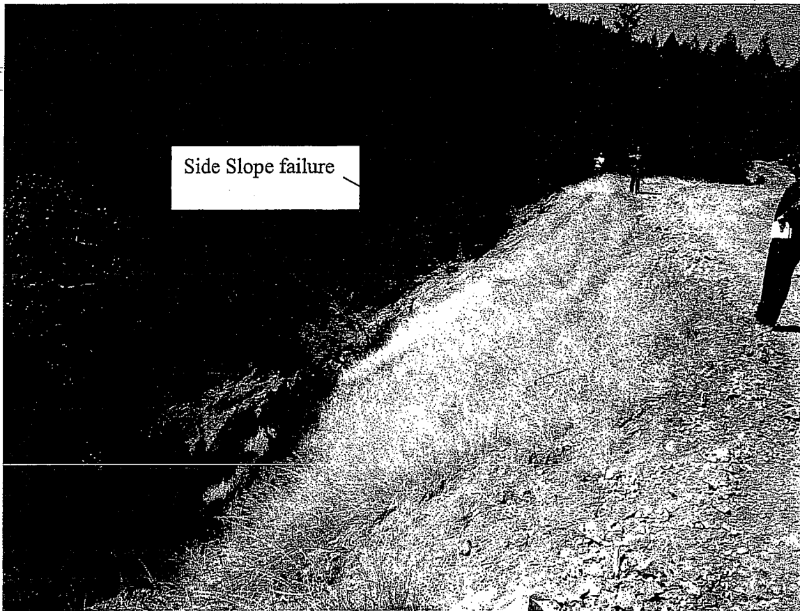
9/25/2009 This photo is taken at the top of the previous road fill failure and shows the side slope failure integrating into the debris chute. The side slope failure may in part be due to side cast of earthen debris during road construction.
