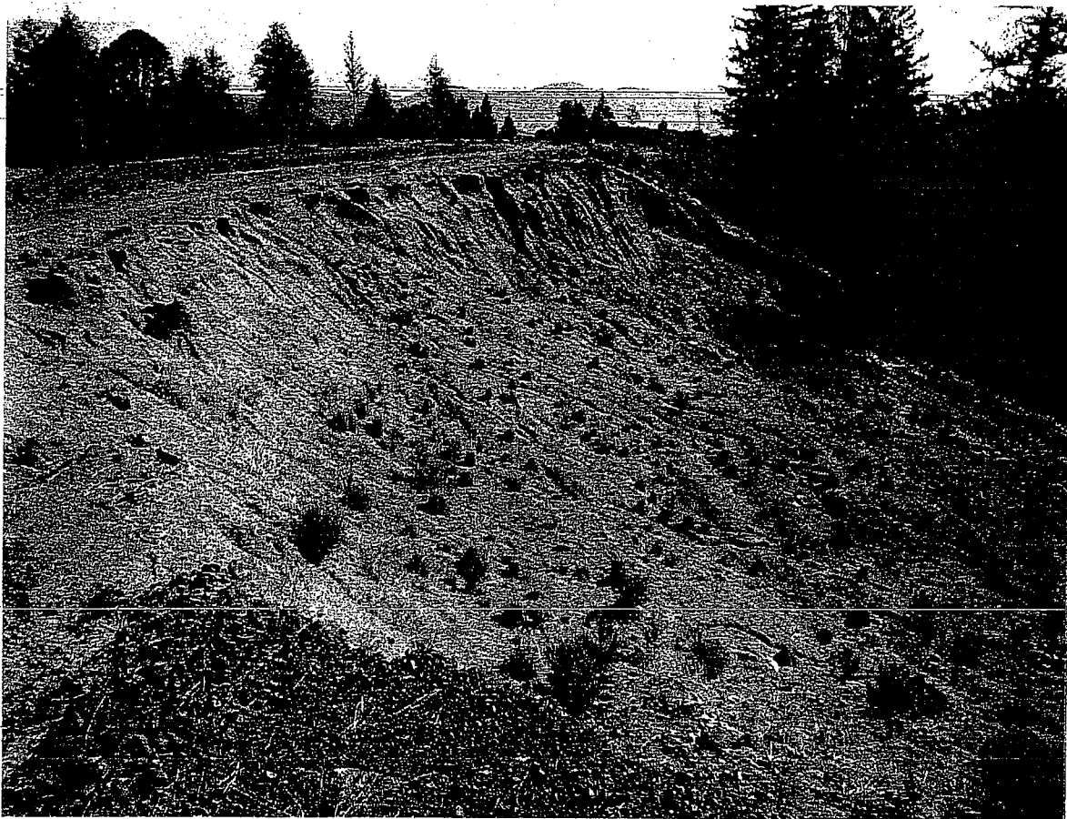
10/17/2008 Upper extent of Site 8 failure
