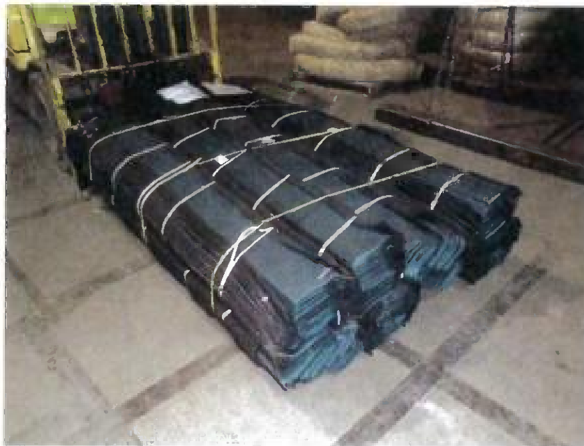
Ertec™ stormwater filtration barrier awaiting installation along edges of concrete dock. Expected project completion – October 31, 2012.
