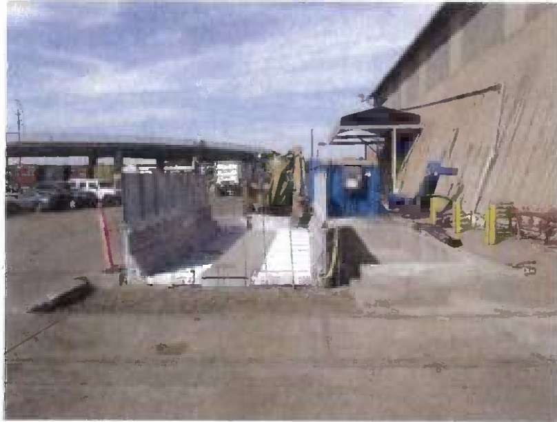
Construction project underway to install commercial wheel washing station at facility exit. Expected project completion – October 1, 2012.
