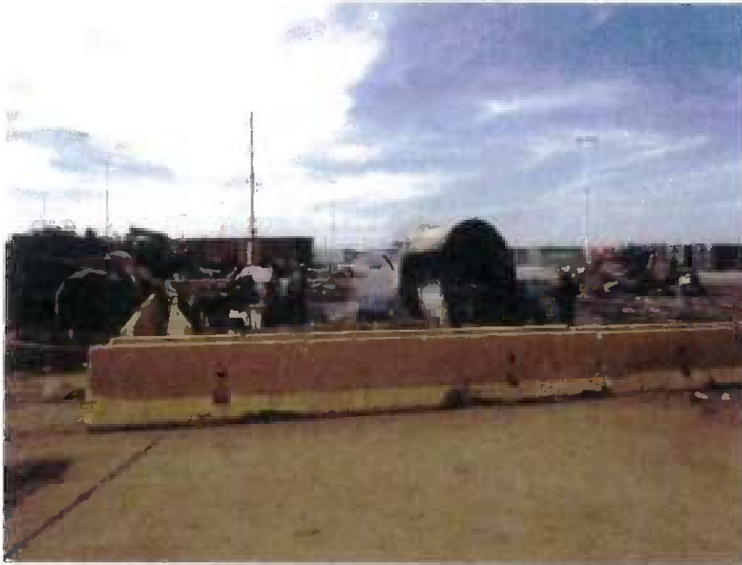
Torch-cutting station relocated to paved and contained area. Project completed – June 2012.
