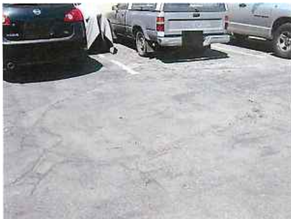
FIGURE 1 – Possible former drywell location in southwest area of parking lot (Pit 3).
