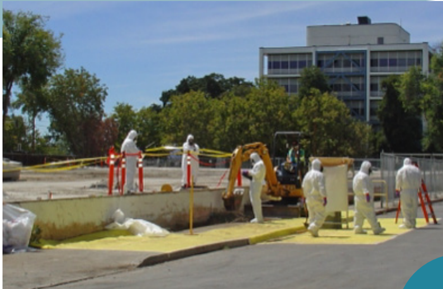
Photo to right: Removal of mercury from soil at Lawrence Livermore National Laboratory, a DoE site
