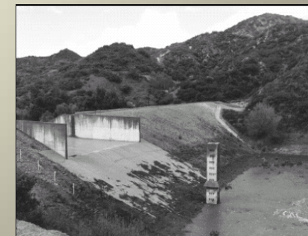
Plate 7.1 The La Tuna Canyon debris basin (Photograph courtesy of K. Barzou)
