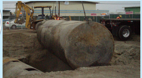
A&P Gas During UST Removal
