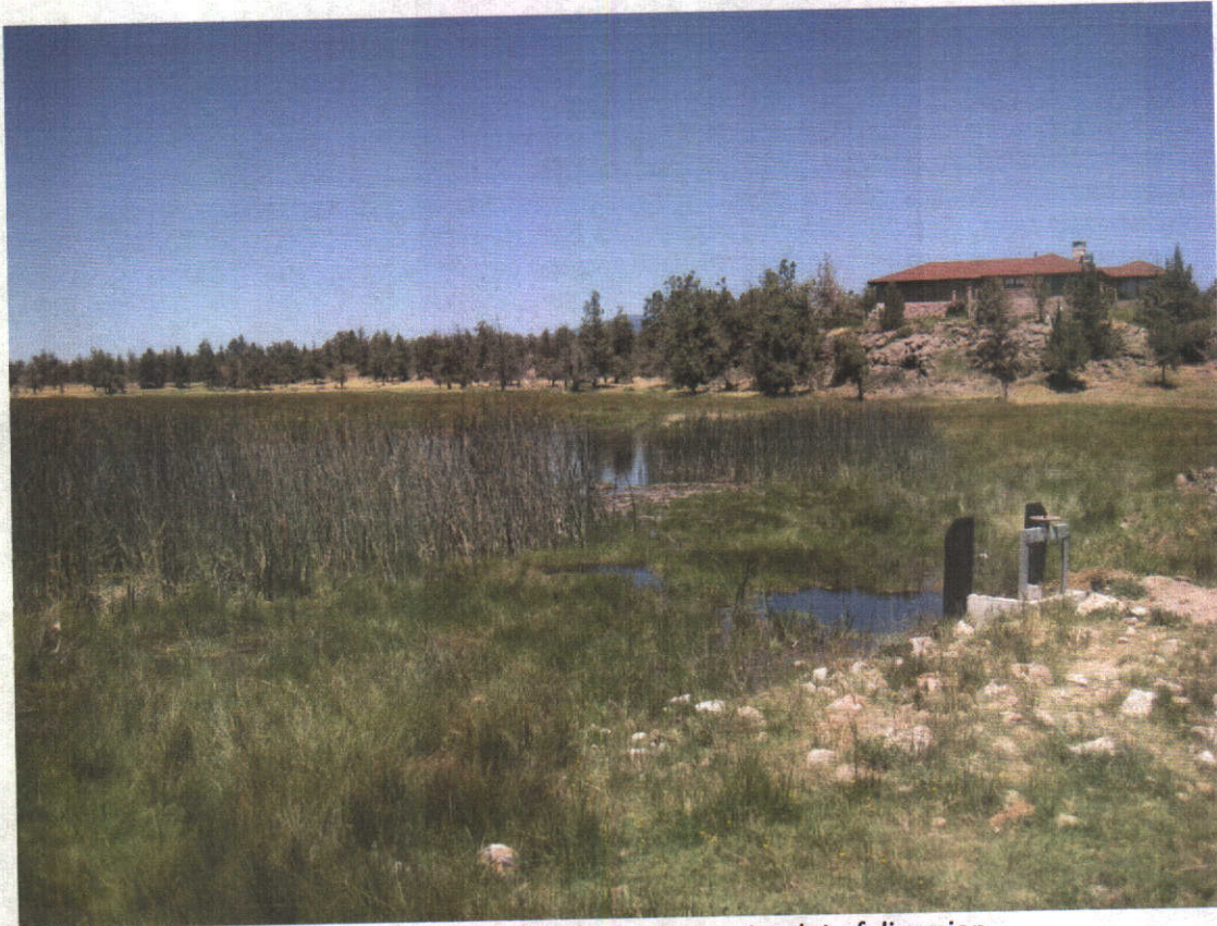
Photo 1 : Diversion #243 Looking immediately upstream at point of diversion. Date Taken: 6/19/2012
