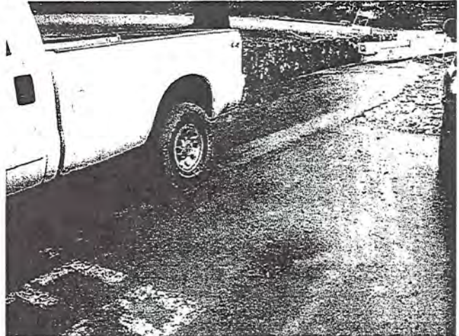
Photo 4. View of a vehicle leaving the construction area with muddy tires.
