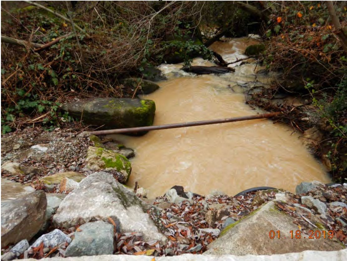
Photo 9. Water in Secret Ravine tributary downstream from Project's dewatering activities.
