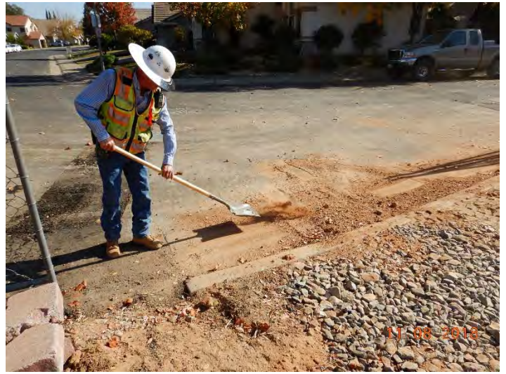
Photo 8. Construction crewmember removing sediment from gutter flow line.
