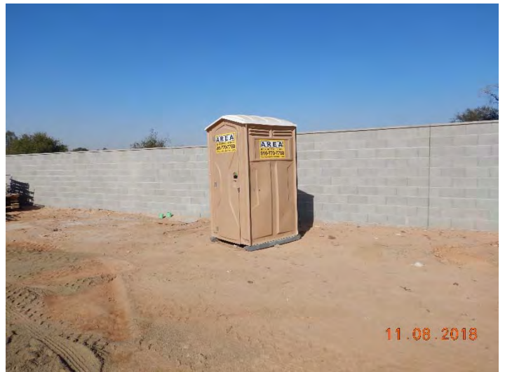
Photo 4. Sanitary facility missing secondary containment.
