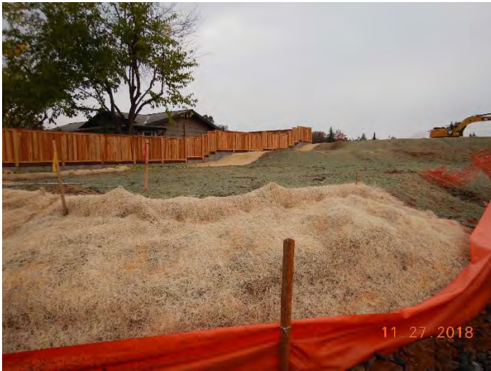
Photo 1. Erosion and sediment control BMPs in inactive areas.
