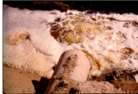
Figure 5. Discharge of Tailwater to Ag Drain.
