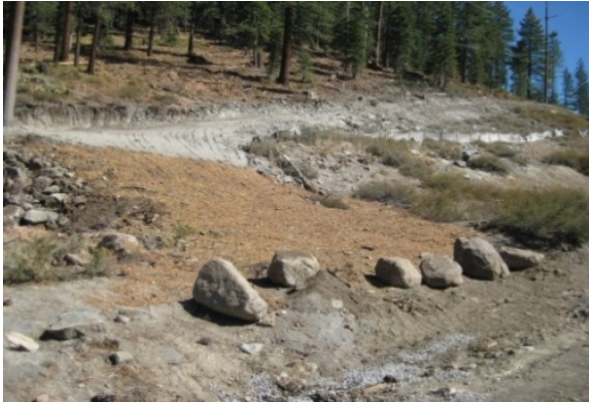
Photo taken on October 5, 2016 prior to placement of Water Board required temporary BMPs to prevent soil from leaving the construction area.
