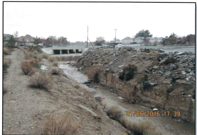
Photo 1 – View looking upstream in Oro Grande Wash towards Seneca Road box culvert crossing during a moderate storm event in January 2016. Downstream of the crossing, the bed of the channel has eroded up to 15-feet over last 20 years.
