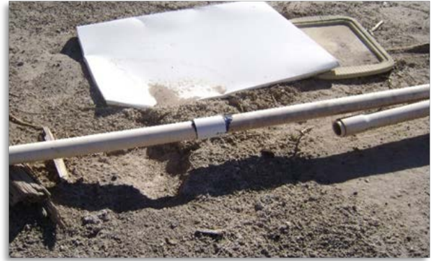
Figure 3 - Broken pipe repaired
