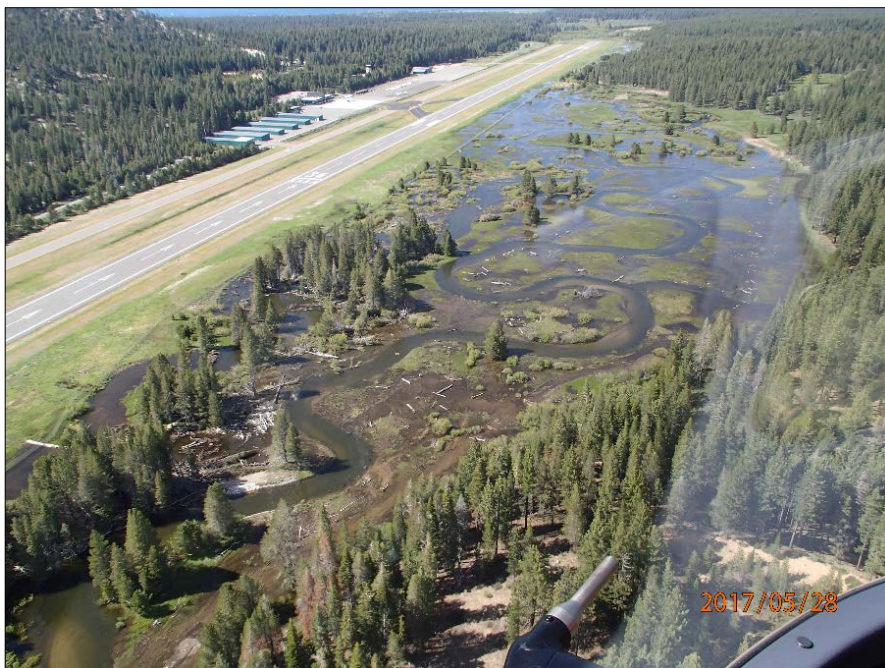
Photo 1: Upper Truckee River Project over-bank river flows in late May 2017. The partially backfilled historic channel can be seen on the left side of the meadow nearest the airport runway, and the newly constructed channel is visible in the middle of the meadow. The goal of area with the project is to re-connect the river with its floodplain, which is evident in this photo showing much of the meadow flooded.
