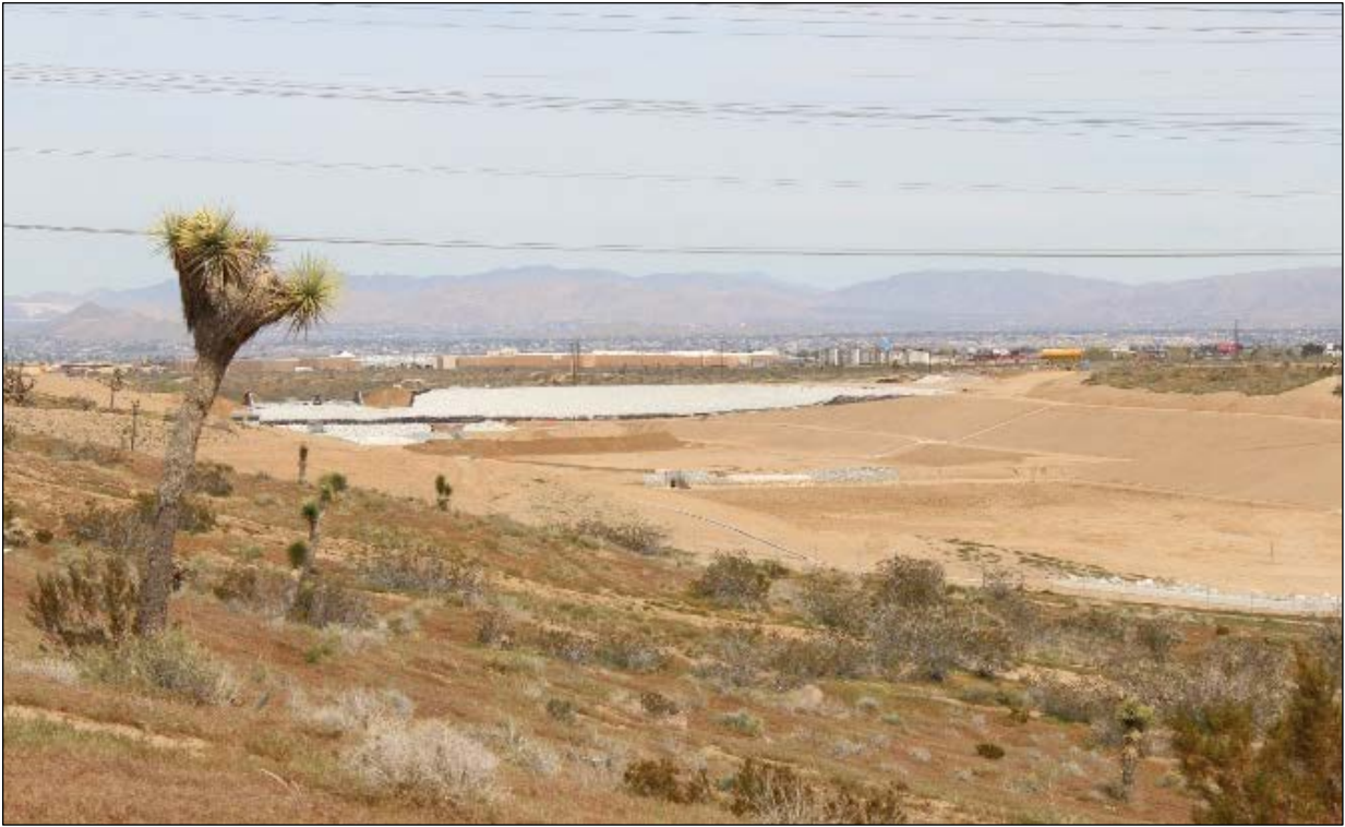
Figure 11a - View of Amethyst Basin with dam and spillway in the background.
