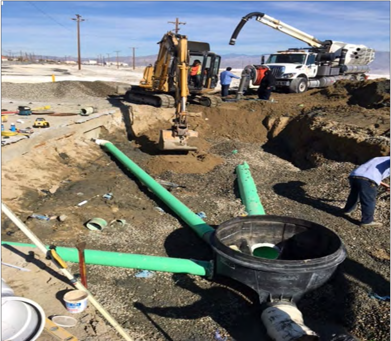
Figure 9.5 - Project to restore flow in the effluent outfall pipeline after earthquake changed infrastructure elevations.
