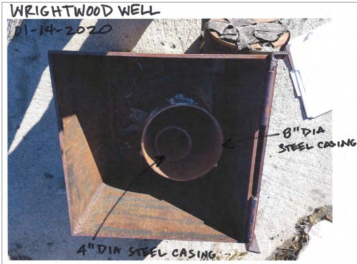
Figure 13.5 - Former San Bernardino County Services Area (CSA) 56 monitoring well. There is no secured cover. The steel casing is not secured and locked and the steel box cover is not secured to.
