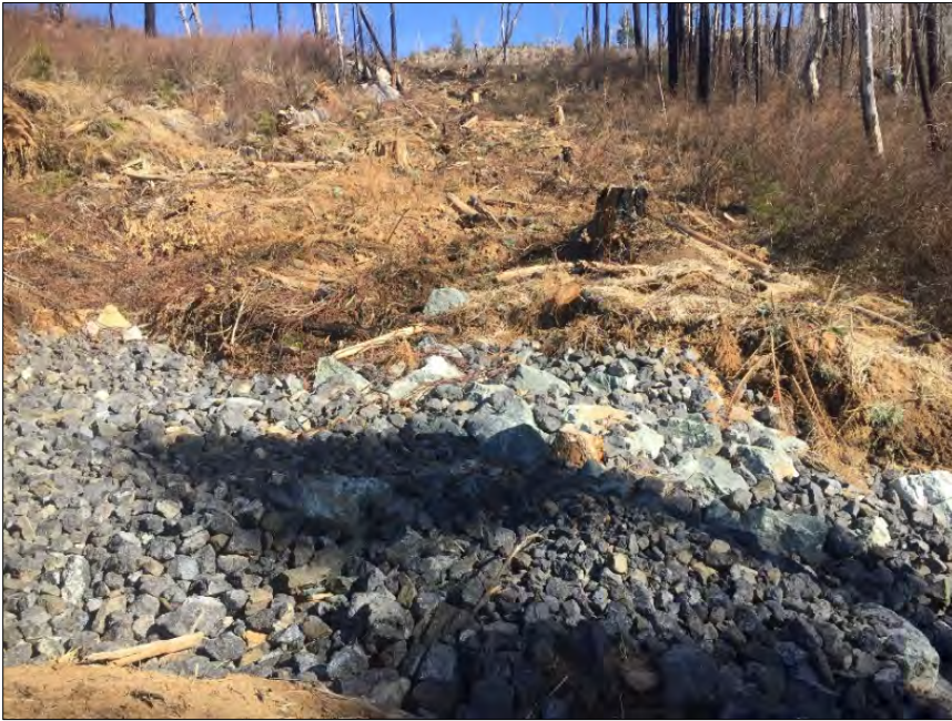
Figure 5.4 - Creek hillside damaged from timber harvesting equipment. Rock fill was used to prevent sediment delivery to the creek below.
