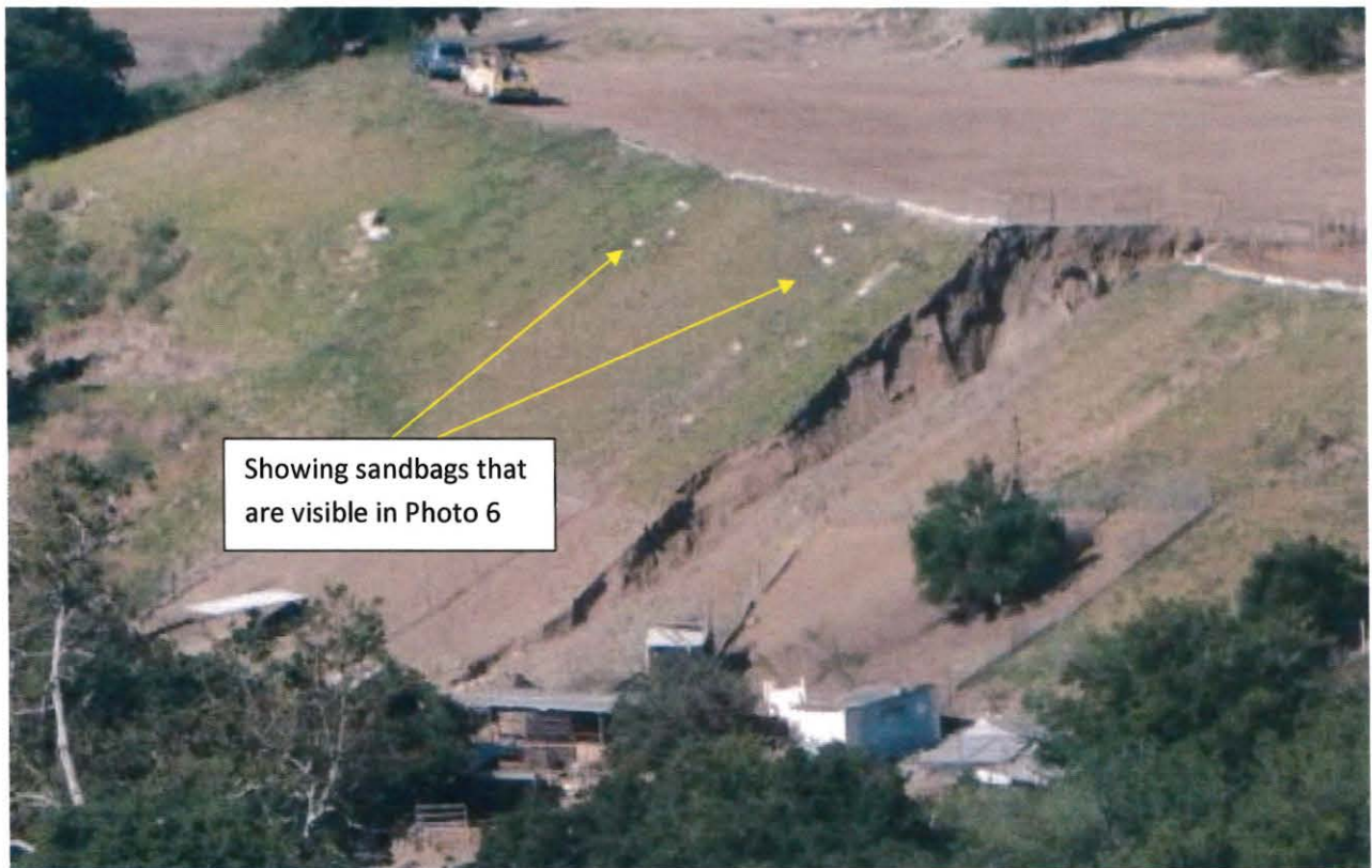
Photo 4. View looking southwest from Photo Location 1. Close up of Photo 3. Showing the sandbags from the sandbag wall that have fallen down the fill slope. These sandbags are visible in Photo 6 and were present during the October 17, 2016 Inspection.
