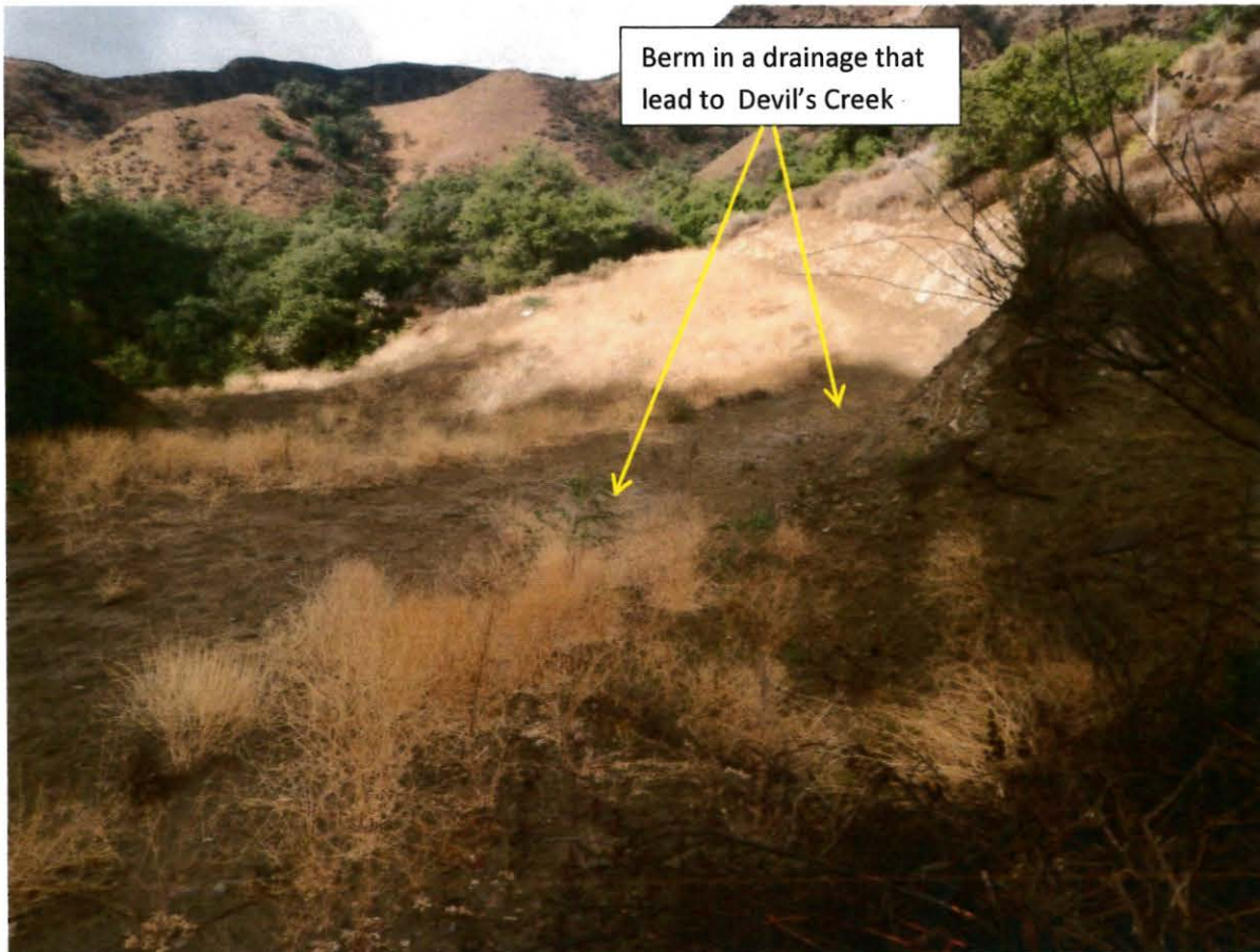
Photo 3. This photo shows another view of the berm in drainage that lead to Devil's Creek that was also shown in Photo 2. This photo was taken in Parcel 2821-002-025 at latitude: 34 18.729 and longitude: -118 37.367.
