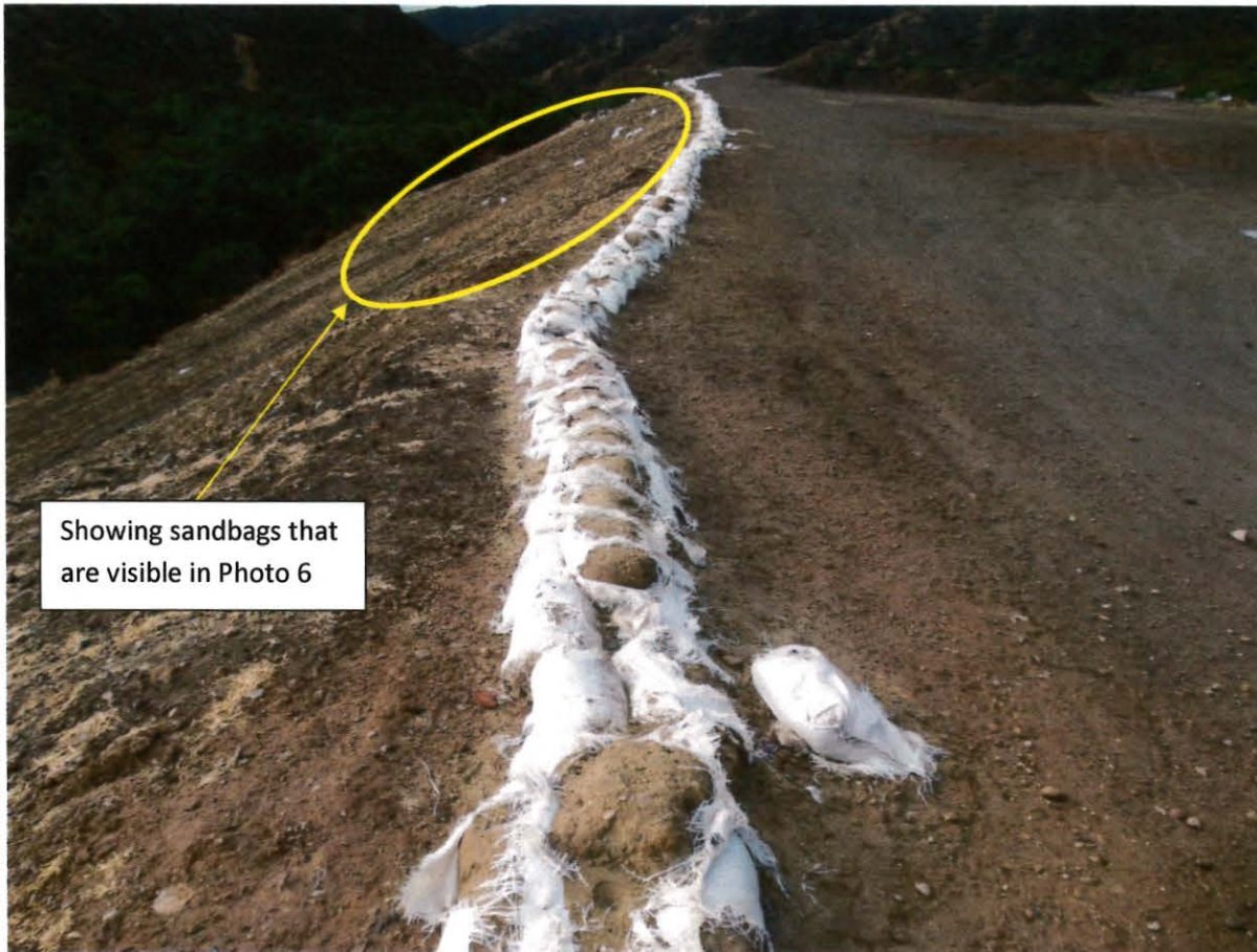
Photo 6. Close up of the sandbag wall along the slope break of the fill slope in Photos 3 and 4 during the October 17, 2016 inspection. The sandbag wall is above the large erosional scour that later developed during the February 2017 rainstorms. The photo shows that number sandbags from the sandbag wall have already fallen down the fill slope. The photo also shows that the sandbags, as of October 17, 2016, were deteriorated and releasing sediment so that they could not function as an effective best management practice (BMP) for subsequent winter storms.
