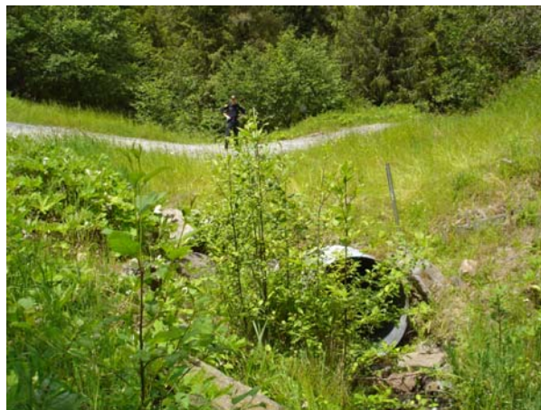
Figure 36. John Munn, CDF, at a culverted watercourse crossing in a forested watershed on the North Coast of California without diversion potential. Munn is standing in the critical dip.
