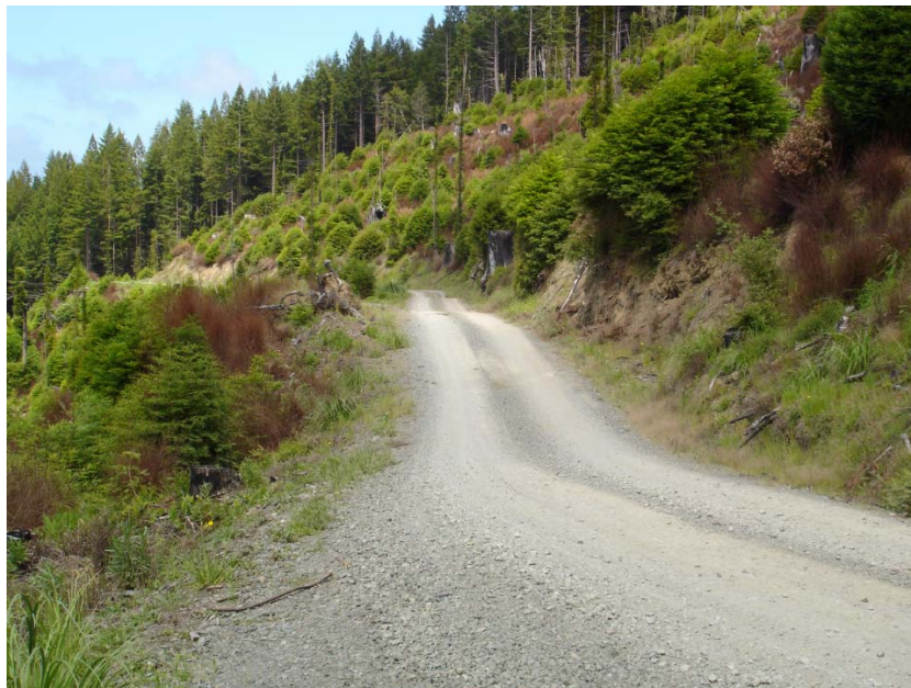
Figure 19. Example of road segment built to drain properly in wet weather. Note the two functional dips and their spacing.
