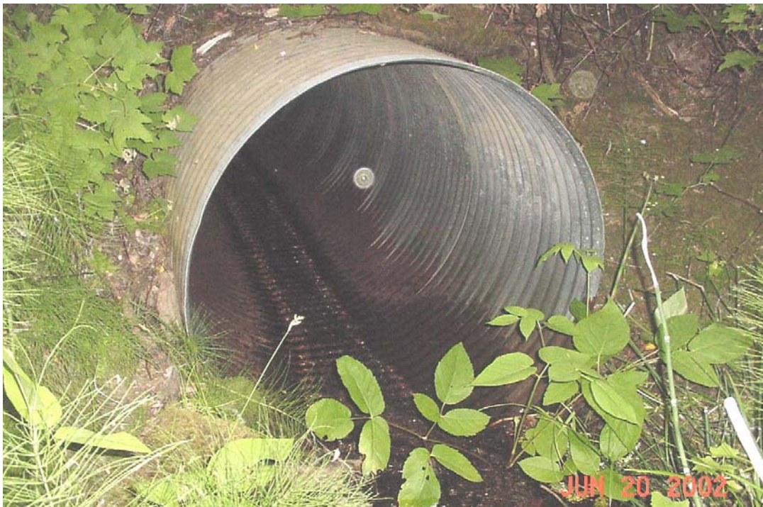
Figure 14. Typical watercourse crossing sampled in the Hillslope Monitoring Program. This culvert was a crossing included in the sample for the 2002 field season.
