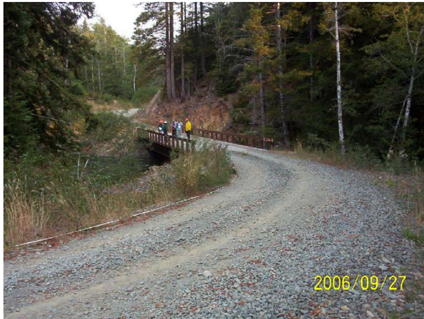
Figure 9. Bridge evaluated in Humboldt County by the Coast team during the 2006 field season. Note the tape stretched along the road approach to measure road length in the WLPZ.
