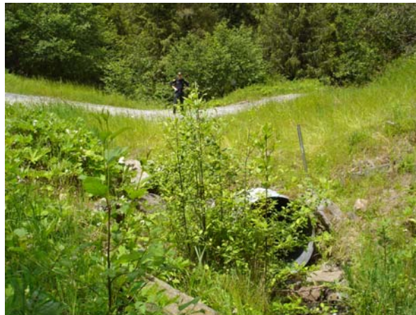
Figure 36. John Munn, CDF, at a culverted watercourse crossing in a forested watershed on the North Coast of California without diversion potential. Munn is standing in the critical dip.
