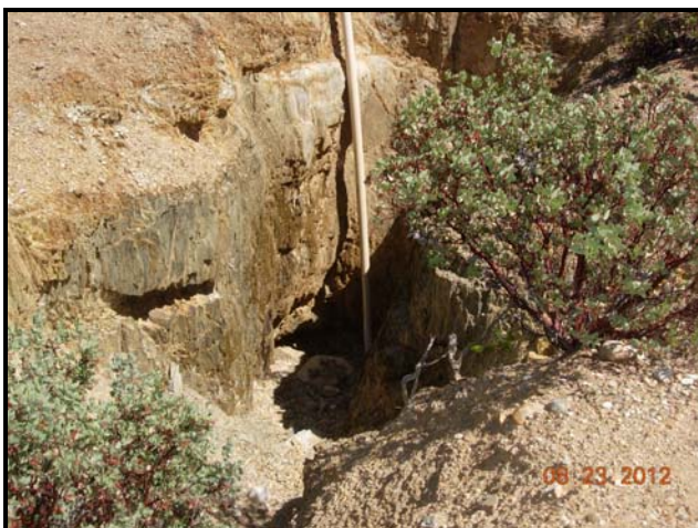
Photo 15. Showing what appears to be a bedrock drain tunnel inlet for discharging mining waste. Further investigation is needed to determine if it's open and if it discharges.
