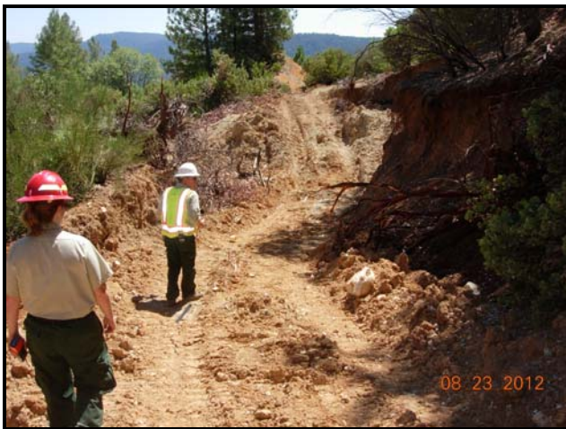
Photo 8. Showing mining waste placed as unconsolidated fill across a ravine.
