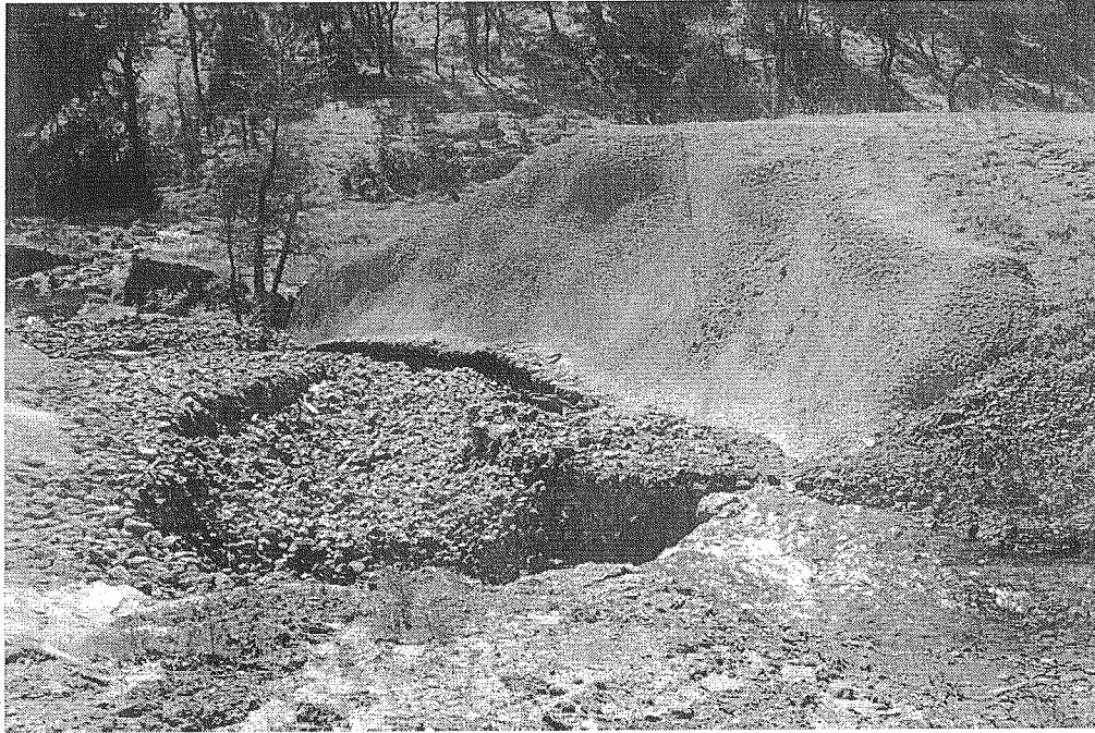
Photograph 1: Before Repair Work
