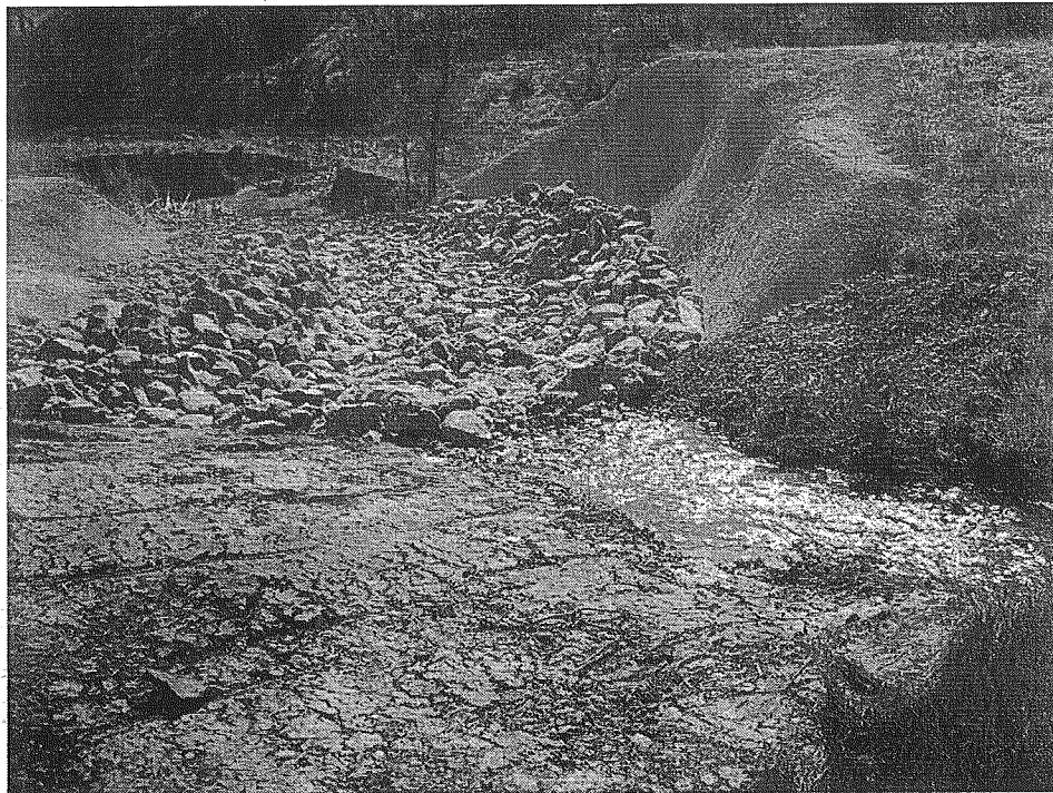
Photograph 2: After Repair Work
