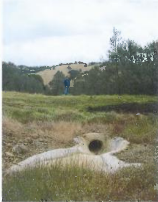
Photograph B-40: Storm water runoff outlet piping from upper mine workings area.
