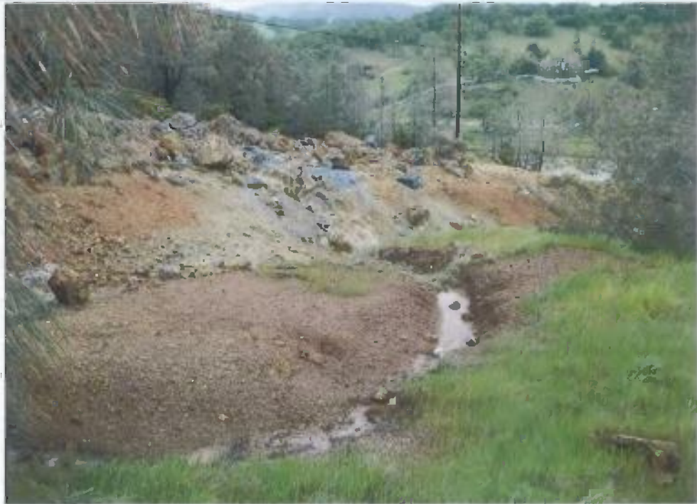
Photograph B-10: Runoff from upper Bradley tailing piles (sample location SW-02).
