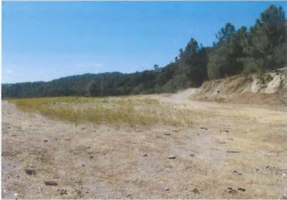
Photograph B-1: Capped area located at the top area of the Bradley tailings piles and waste rock.
