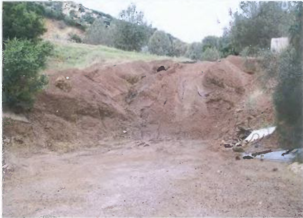
Photograph B-26: Calcine tailings above upper pond area. Drains to upper pond.
