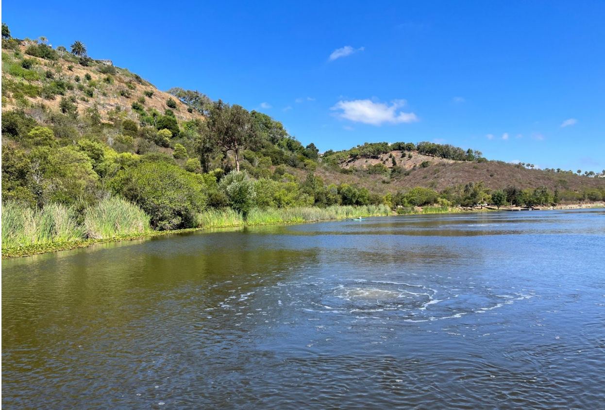
Image: South end of Lake San Marcos showing bubbling at the surface from diffusers installed as part of the Phase I aeration system.
