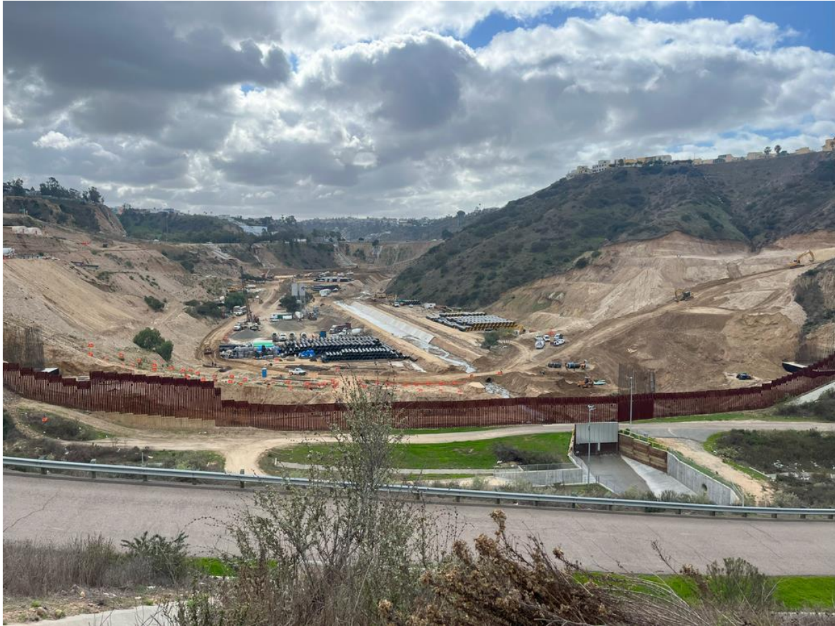
Figure 10: Mexican construction project in Matadero Canyon. (MC 01/10/2024)
