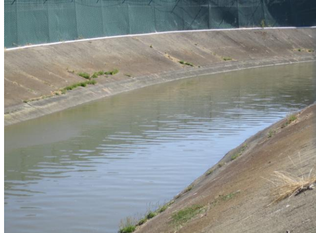
Section of Millbrae Canal that will be placed in culvert
