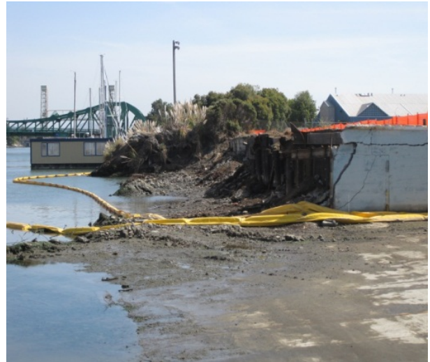
Photo 2 (before) and 3 (after). Collapsed pier removed from the estuary near the intersection of Clement Avenue and Oak Street in Alameda (Courtesy USEPA staff).
