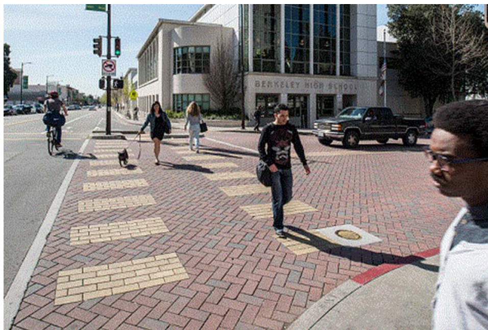
Figure 2. Permeable pavement at Allston Way, Berkeley
