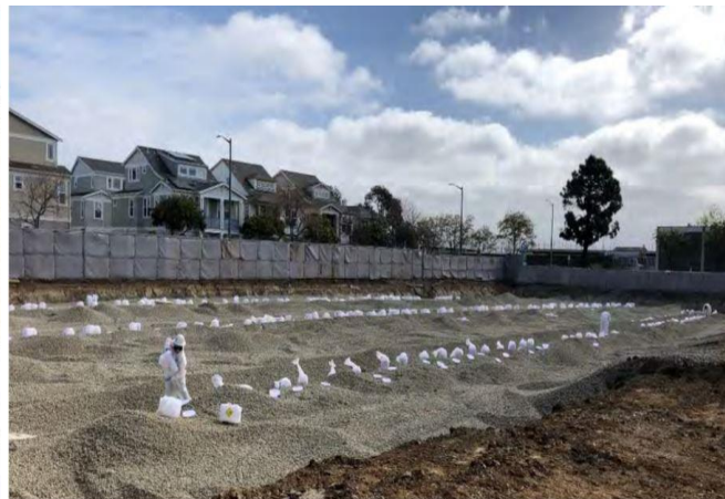
Figures 5 and 6: Excavation and backfill with gravel and ORC application in the northeast portion of the site.
