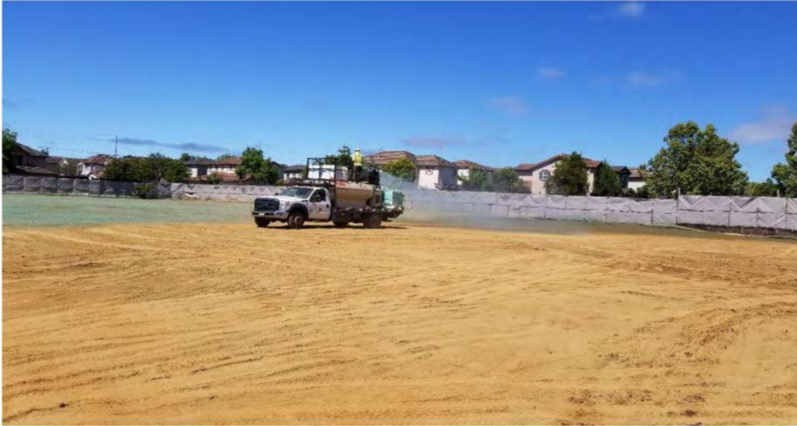
Figure 7: Final grading and hydroseeding after demolition and soil excavation was completed.
