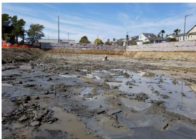
Figures 5 and 6: Excavation and backfill with gravel and ORC application in the northeast portion of the site.
