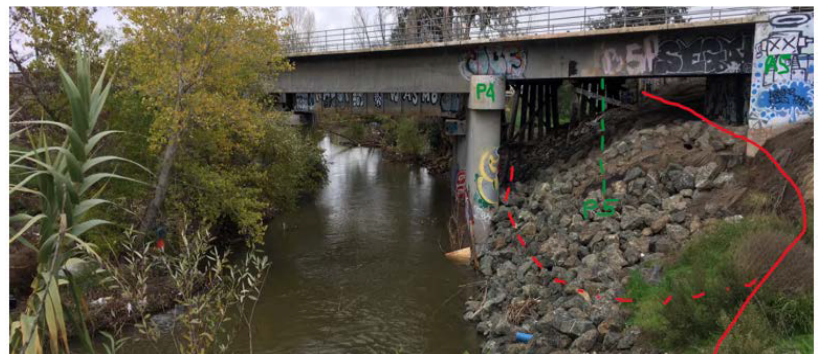
MT2 Bridge – Rock Riprap Stabilization 2017
