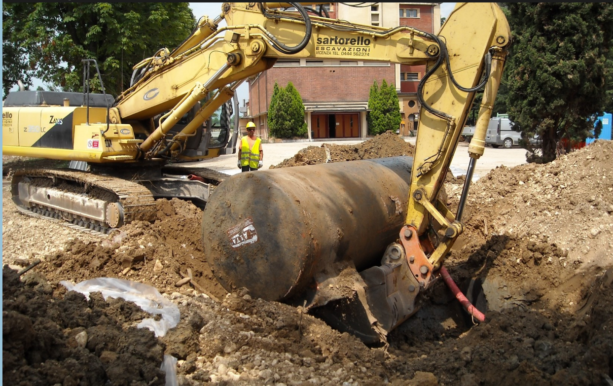
Photograph 1: UST being removed by a backhoe
