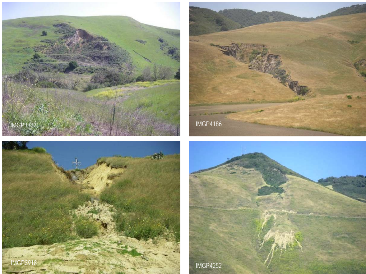
Figure 3-12. Examples of altered watershed processes in response to disturbance. Upper panels, Tertiary deposits express landsliding west of Twitchell Reservoir (left) and gullying south of Guadalupe (right) in response to vegetation changes and soil compaction from grazing; lower panels show effects of concentrated runoff in the form of severe gully-cutting through Quaternary deposits above the Santa Maria River (left) and debris flows below a service road in Franciscan mélange north of Arroyo Grande (right).
