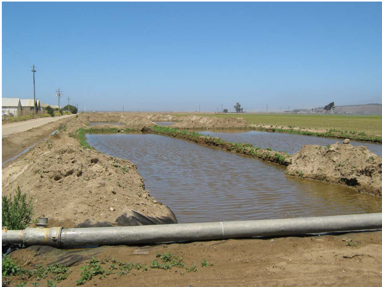
Figure 5-2 A water and sediment control basin at the edge of farm field in the Oso Flaco watershed
