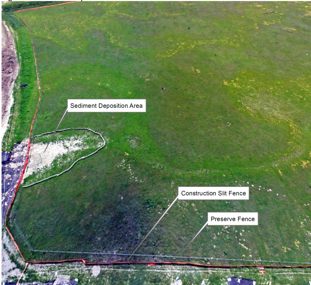
Figure 2: Sediment Deposition in Vernal Pool 167
