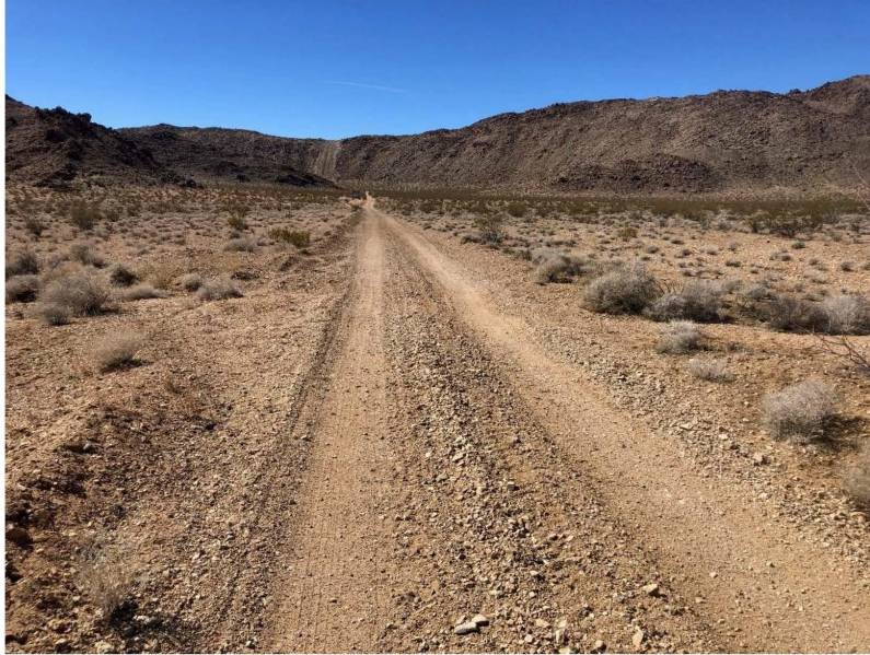
Photograph 3. View of Drainage 1 project area and location of L-4000 pipeline and existing access road (Aspect: West. February 23, 2021).
