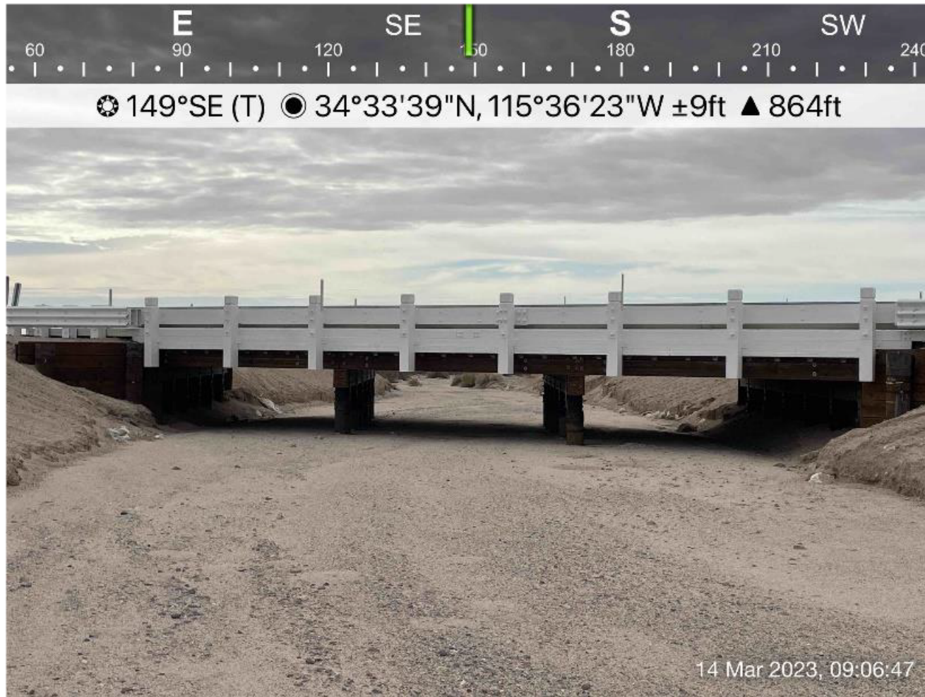
Photo 1: Downstream View of Dola Ditch Bridge, Facing South
