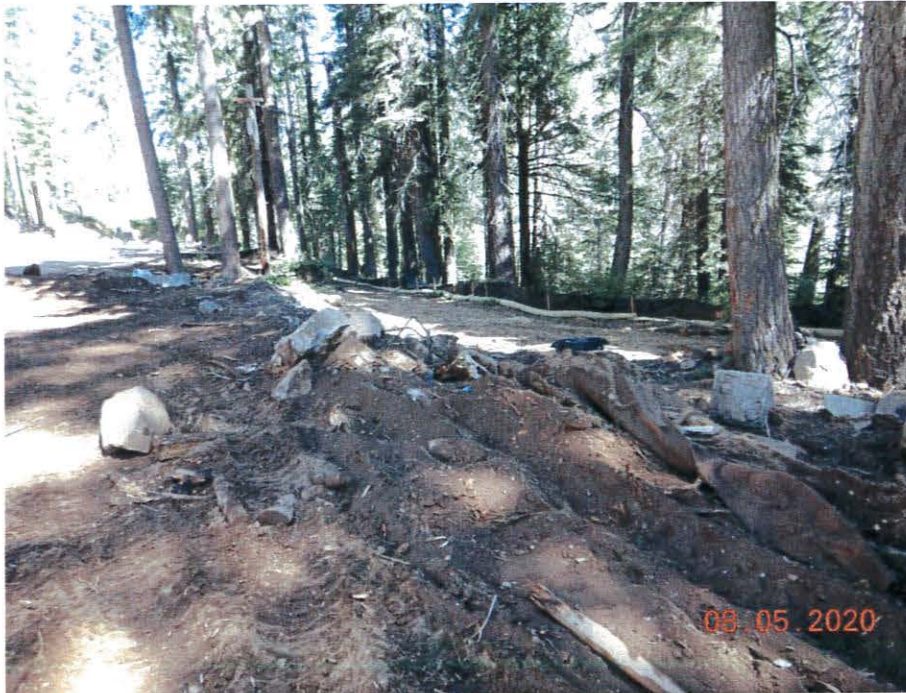
Photo 7. Windrowed soil and rock, downslope perimeter BMPs
