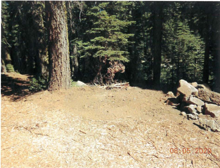
Photo 5. Disturbed soil area partially stabilized with wood chips.
