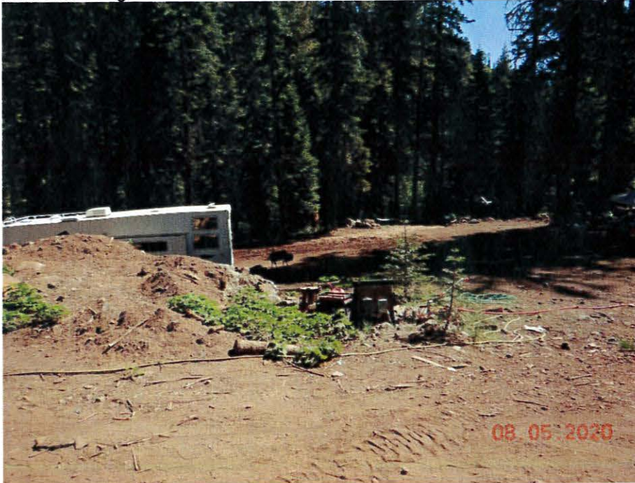
Photo 3. Recently cleared area and stockpiled soil and rock.
