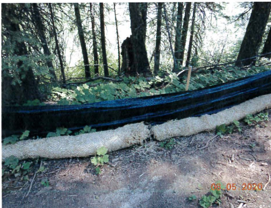
Photo 11. Downslope perimeter sediment control BMPs.
