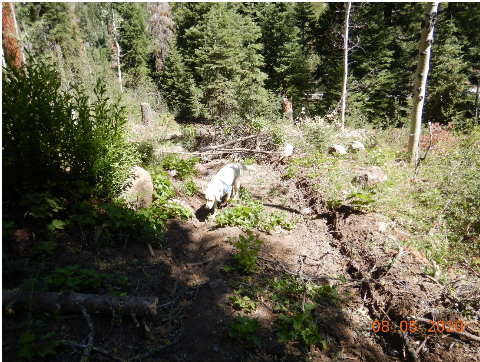
Photo 8. Temporary access road. Ruts resulting from heavy equipment driving on saturated soil.
