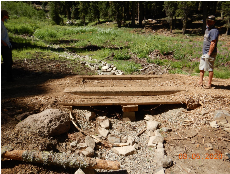
Photo 14: Permanent watercourse crossing.
