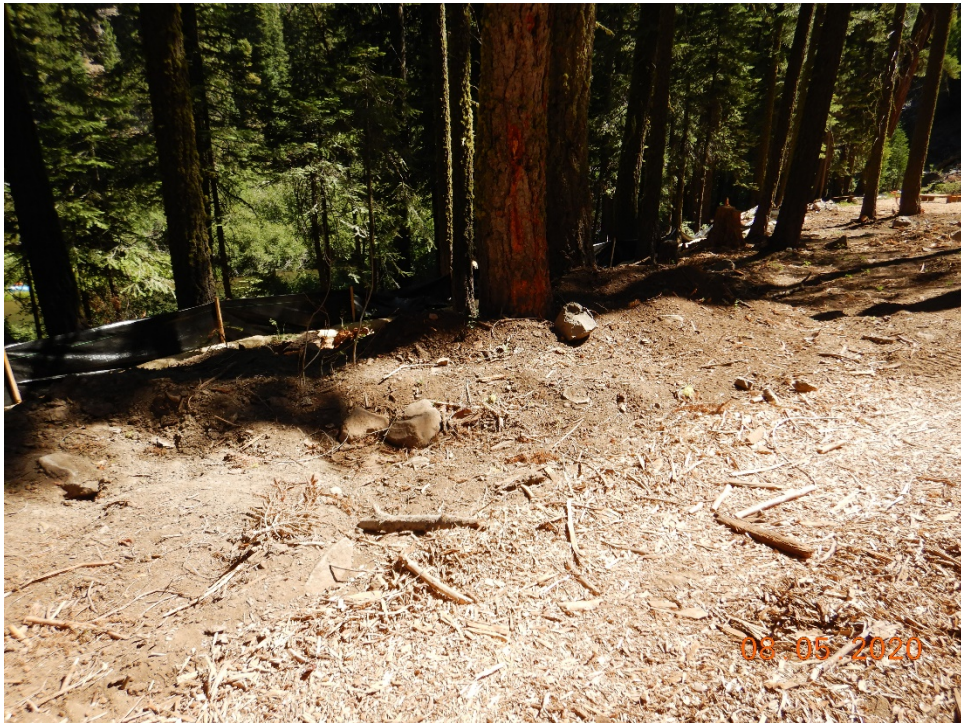
Photo 12. Windrowed soil adjacent to road surface partially stabilized with wood chips.
