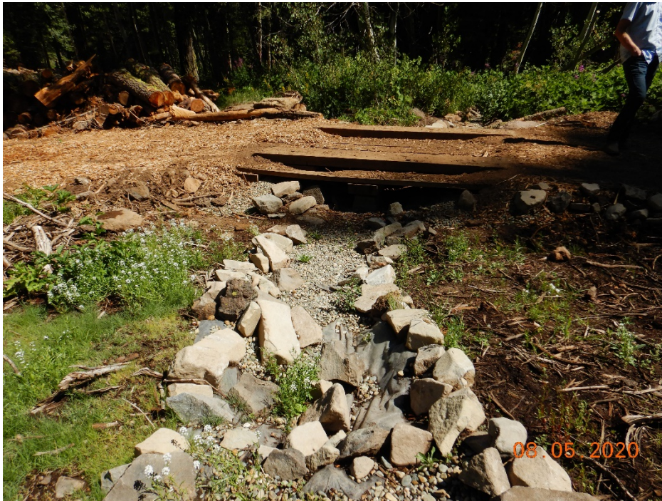
Photo 18. Modified watercourse, permanent watercourse crossing, disturbed soil in SEZ, woody debris and logs stockpiled in SEZ
