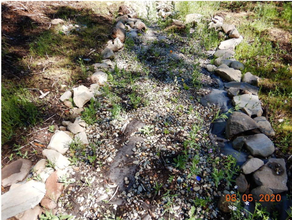
Photo 16. Modified watercourse: straightened, lined with geotextile, covered with gravel, bordered with cobbles.
