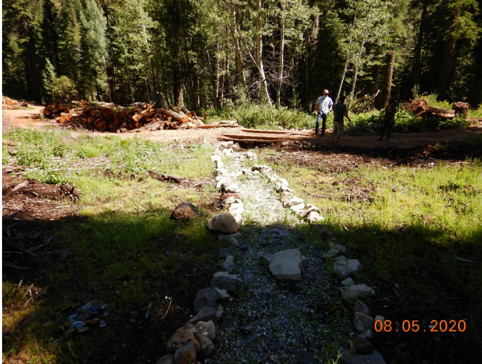
Photo 17. Modified watercourse, permanent watercourse crossing, disturbed soil in SEZ, woody debris and logs stockpiled in SEZ.
