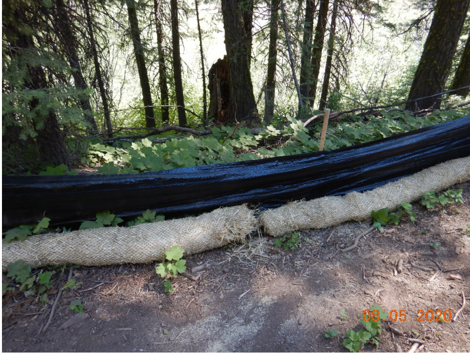
Photo 11. Downslope perimeter sediment control BMPs.
