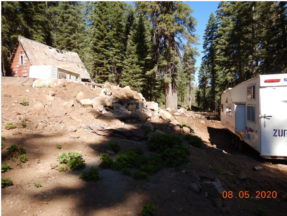
Photo 4. Stockpiled soil and rock.
