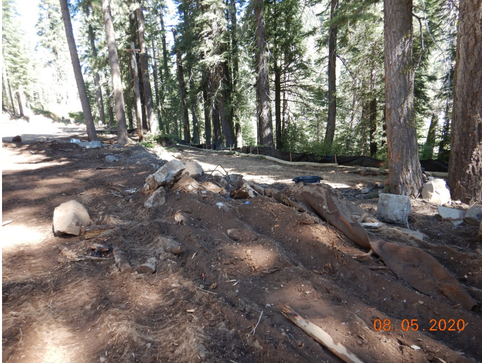
Photo 7. Windrowed soil and rock, downslope perimeter BMPs
