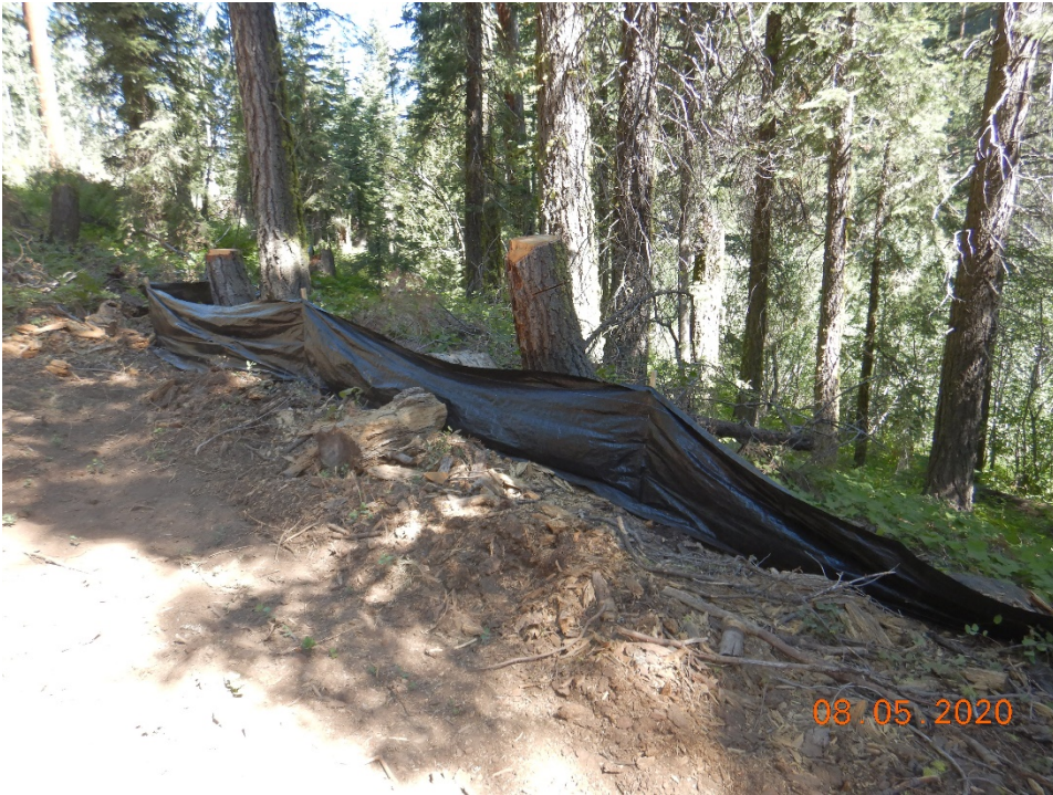
Photo 10. Downslope perimeter sediment control BMP.
