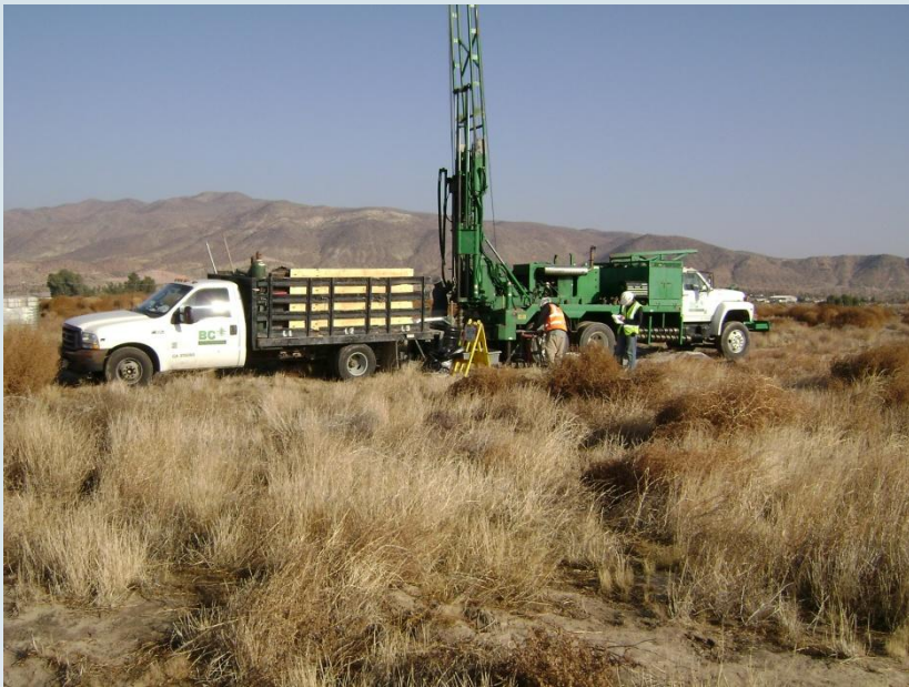
1. Drill to groundwater with hollow-stem auger rig
