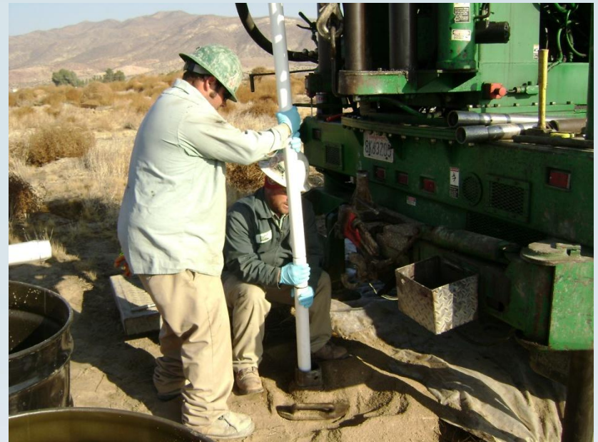
2. Install temporary well casing.
