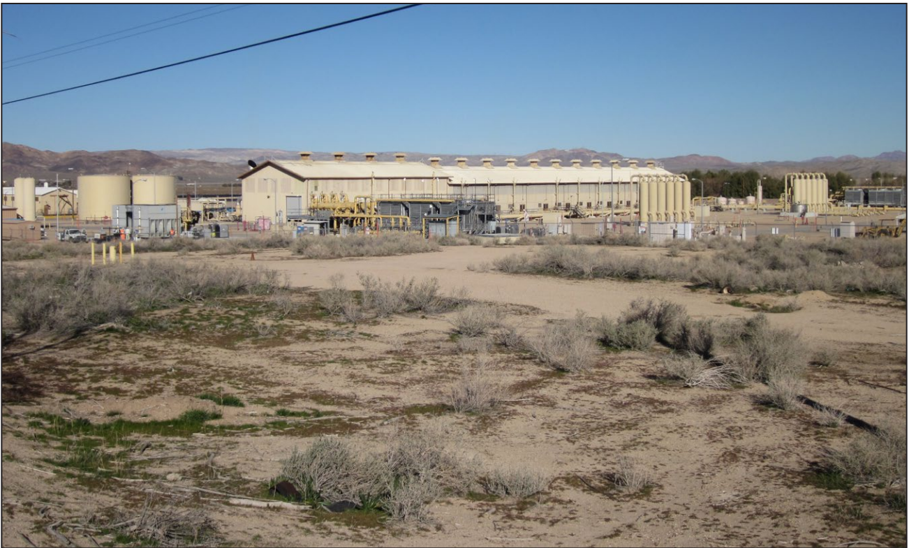
Photo 4: PG&E Compressor Station from Community Boulevard facing southwest (Viewpoint 4).
