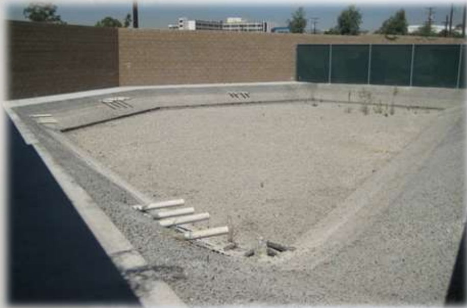
Infiltration Basin Perimeter
