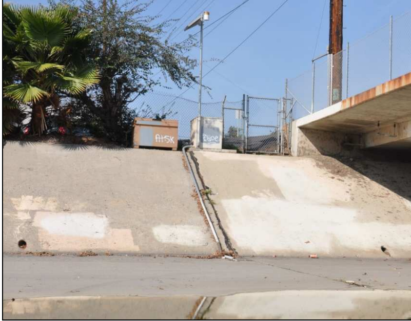
Figure 7: Stearns Street Mass Emission Station
