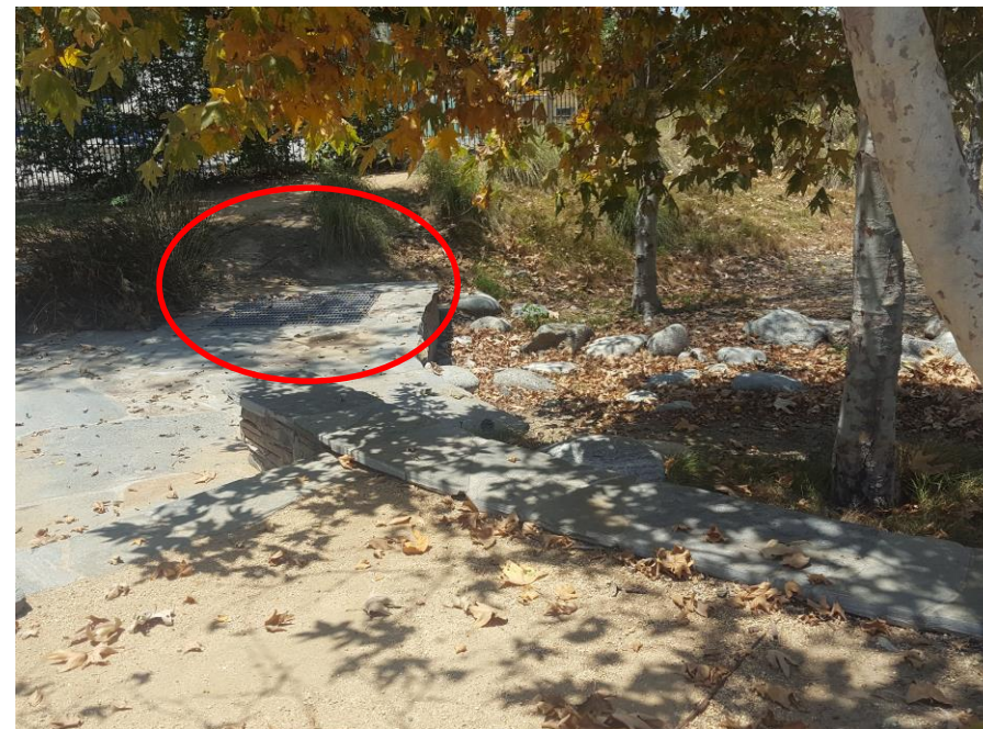
Existing Drainage Basin and Storm Drain Inlet at South End of Park (from NE looking SW)
