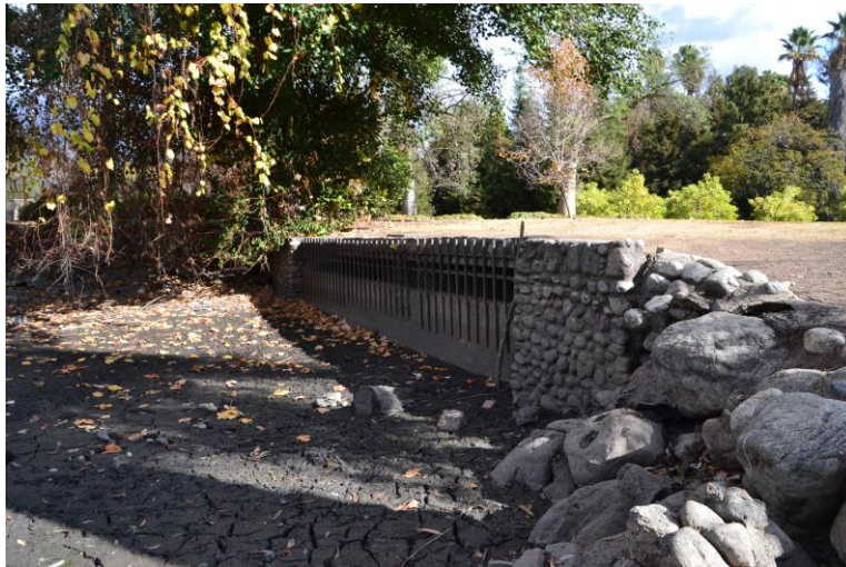
Figure 4. Tule Pond Existing Conditions and Outlet Structure
