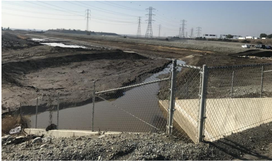
Figure 4. Bradbury Channel Outlet to Basin 3E with Standing Water (Looking from North to South)
