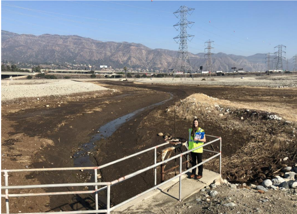
Figure 2. Basin 3E Looking from South (at Gate Valves) to North
