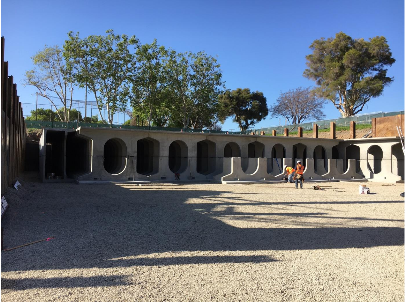
Figure 10. StormTrap Installation ad Bolivar Park BMP
