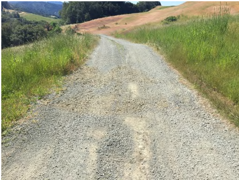
PWA RD1: Gravel patch work to fill shallow depression (May 2017)
