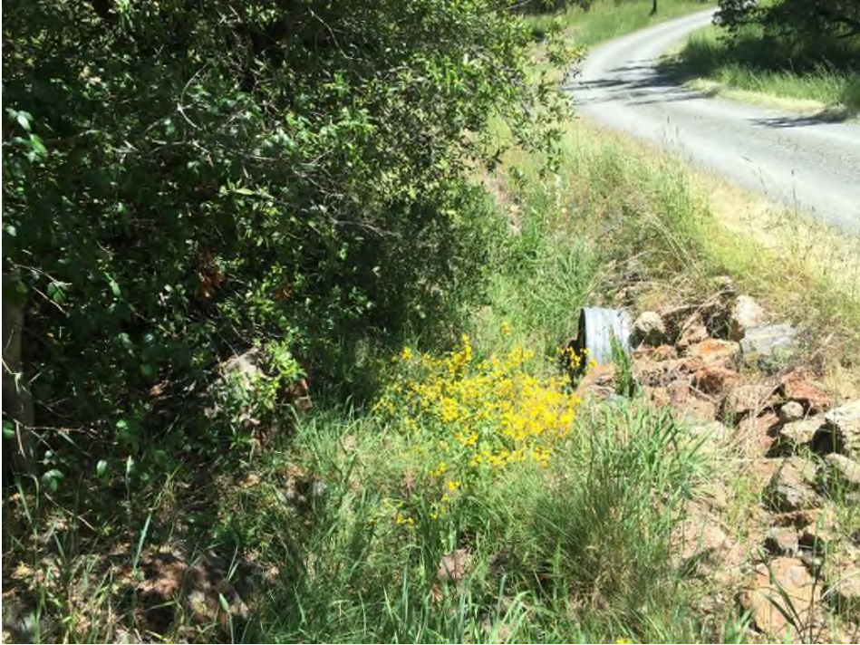
PWA Site #2 (May 2016)
