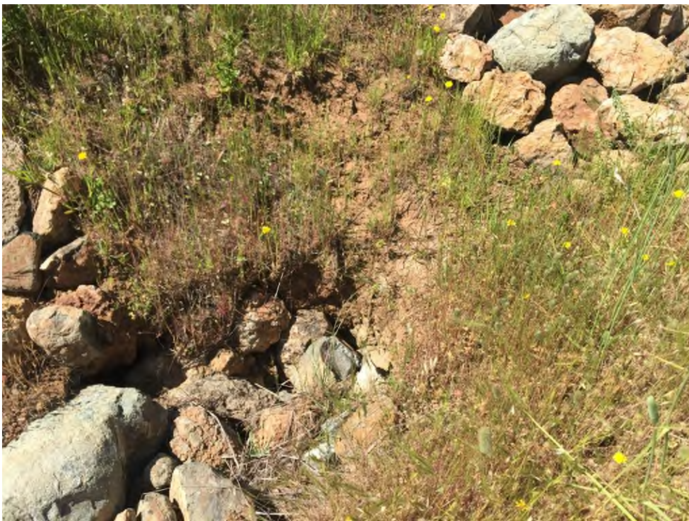
PWA Site #8.1 Rock armor repair at Grade Control Structure Headcut (May 2017)
