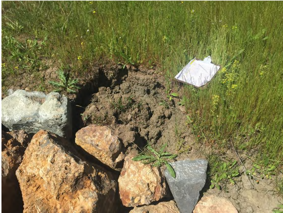
PWA Site 7.2b - Headcut has developed at the top right corner of the rockslope protection (May 2016)
