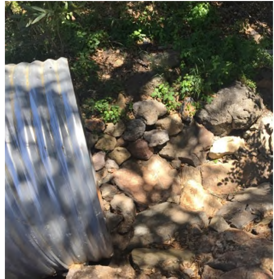
PWA Site #5 scour pool re-rocked (May 2017)
