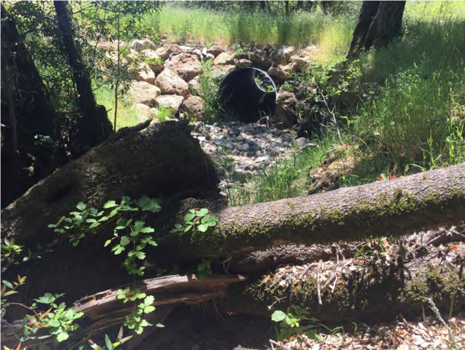
PWA Site #6 inlet (May 2017)
