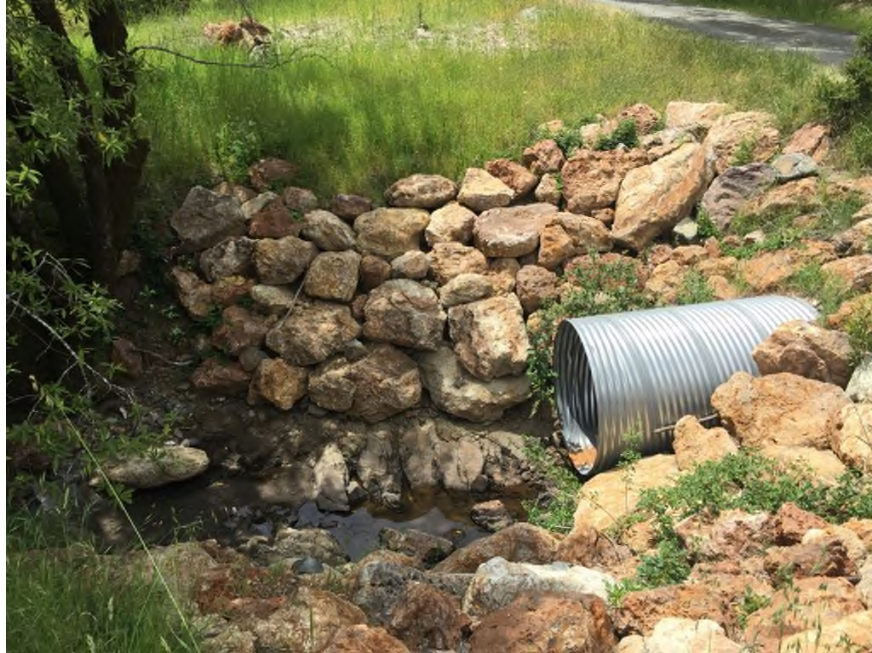
PWA Site #6 outlet (May 2016)
