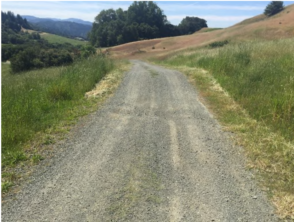
PWA RD1: Shallow depression (May 2016)
