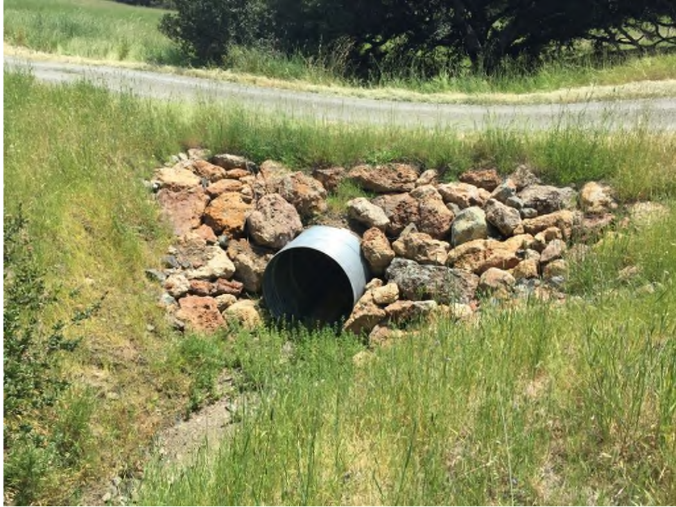
PWA Site #5 inlet (May 2016)
