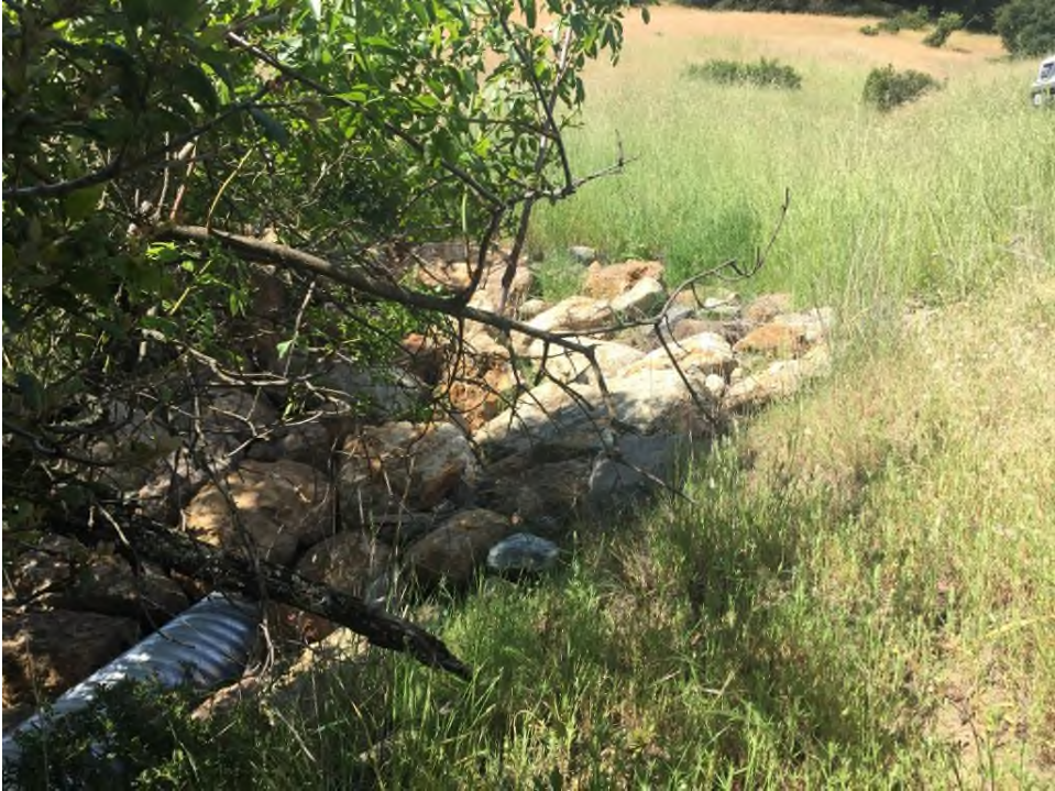
PWA Site #7 (May 2016)
