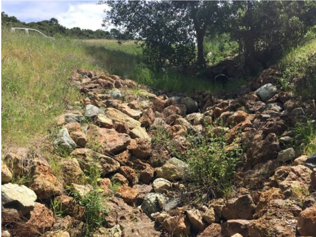
PWA Site #11 (May 2016)
