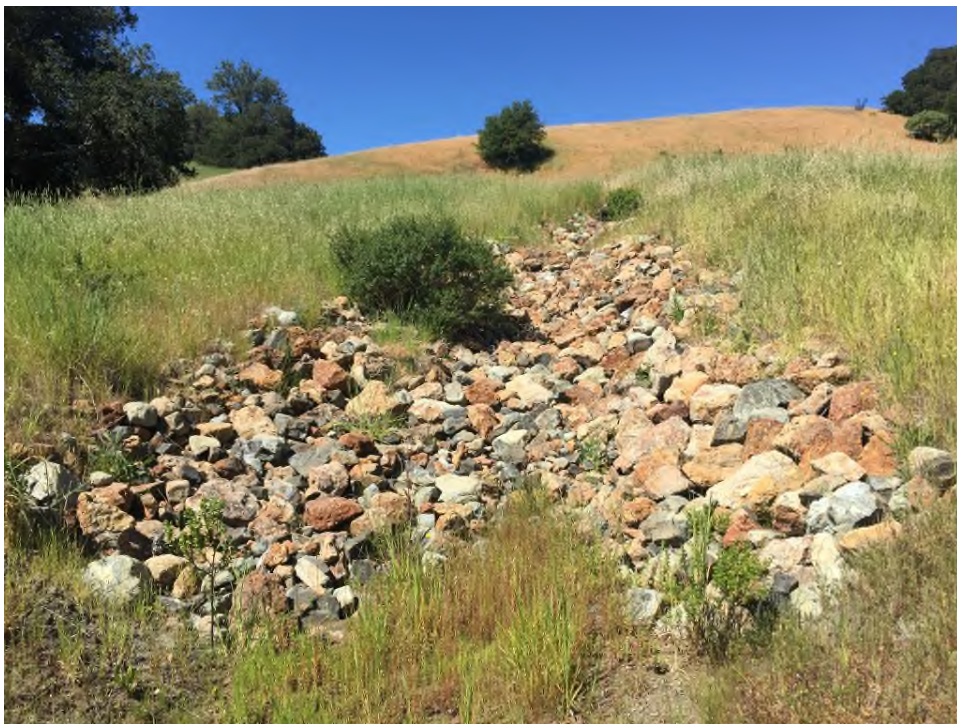
PWA Site # 8.1 (May 2017)
