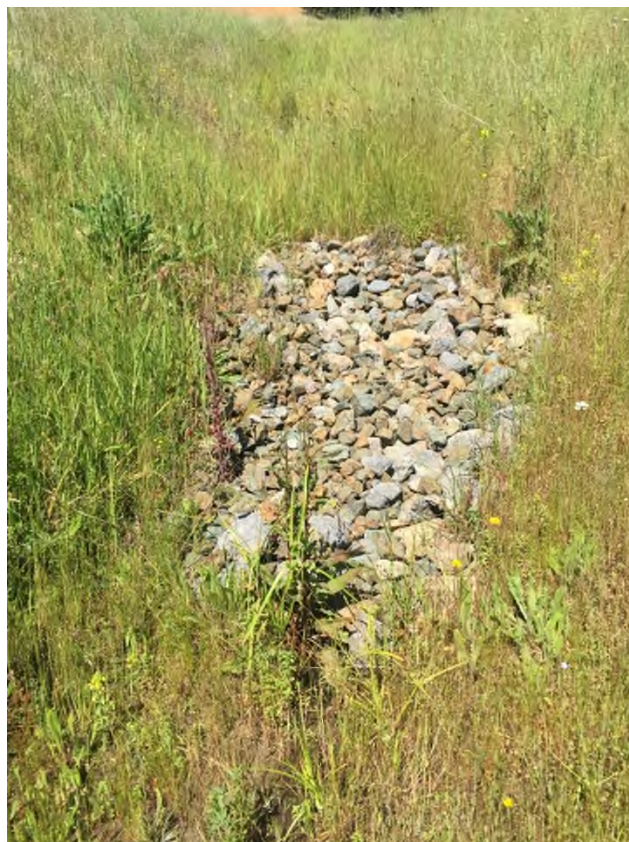
View of rock-armored headcut above PWA Site #6.2, below PWA Site #8.1 (May 2017)
