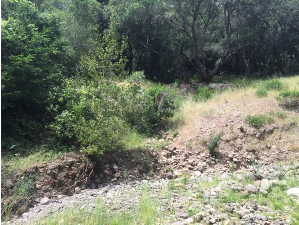
PWA Site # 25 (May 2016)
