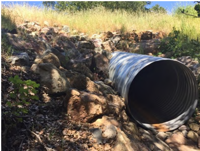
PWA Site #5 outlet (May 2017)
