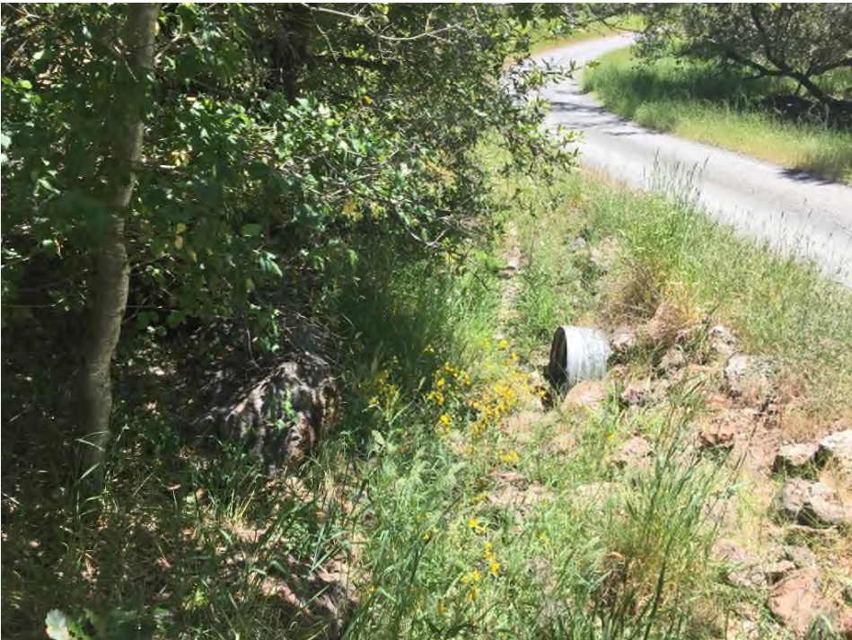
PWA Site #2 (May 2017)
