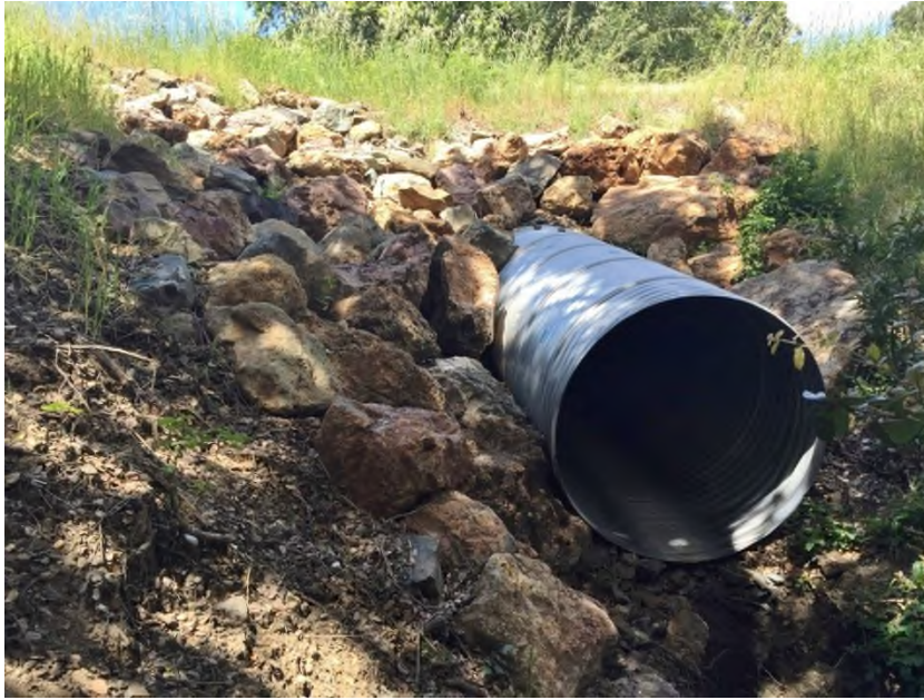
PWA Site #5 outlet (May 2016)
