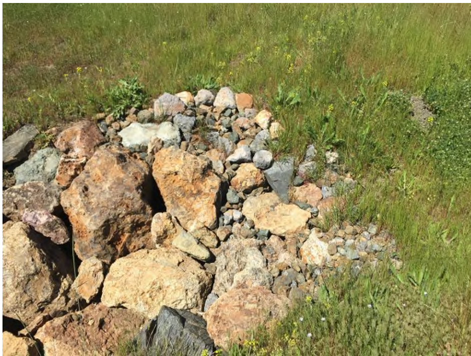
PWA Site 7.2b – Rock armor treatment repair where inboard road ditch drains to rock armor (May 2017)
