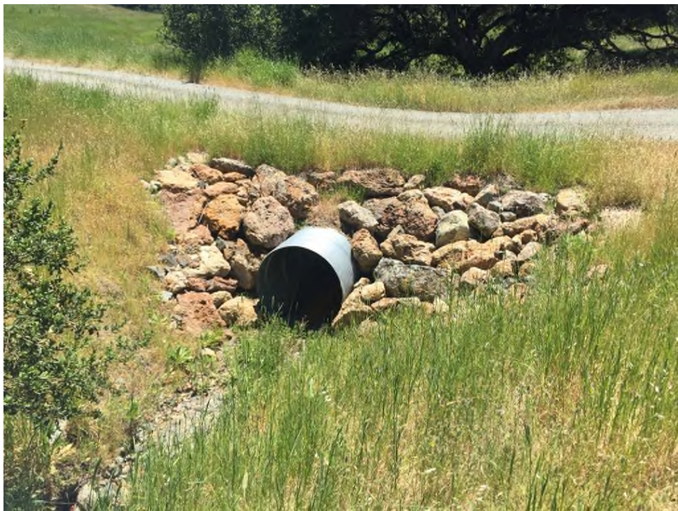
PWA Site #5 inlet (May 2017)
