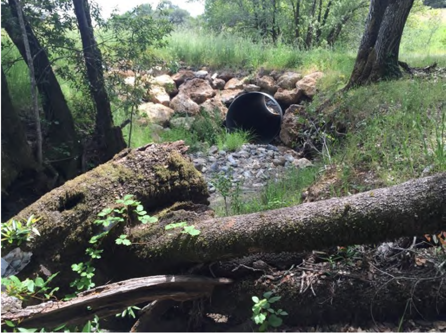
PWA Site #6 inlet (May 2016)
