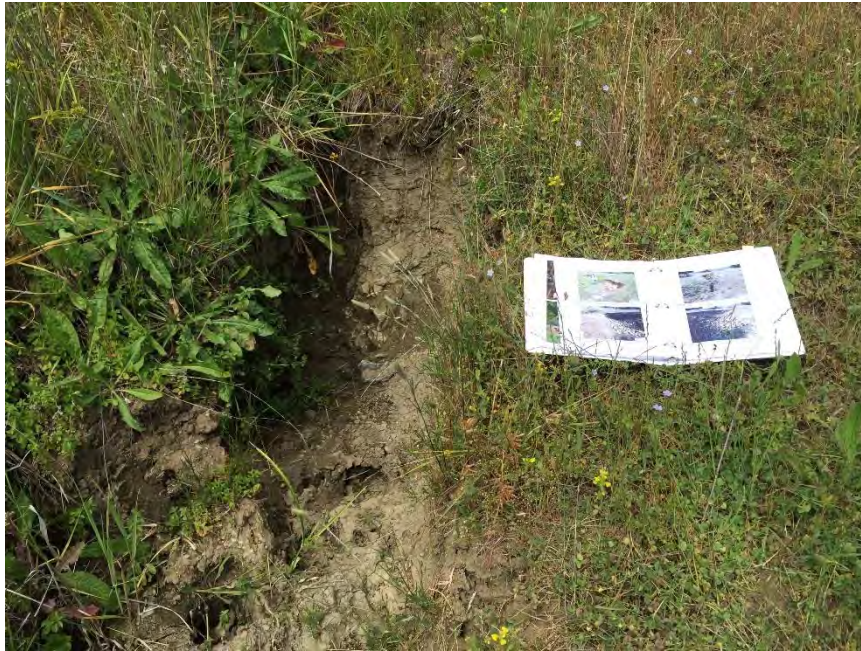
View of headcut above PWA Site #6.2, below PWA Site #8.1 (May 2015)
