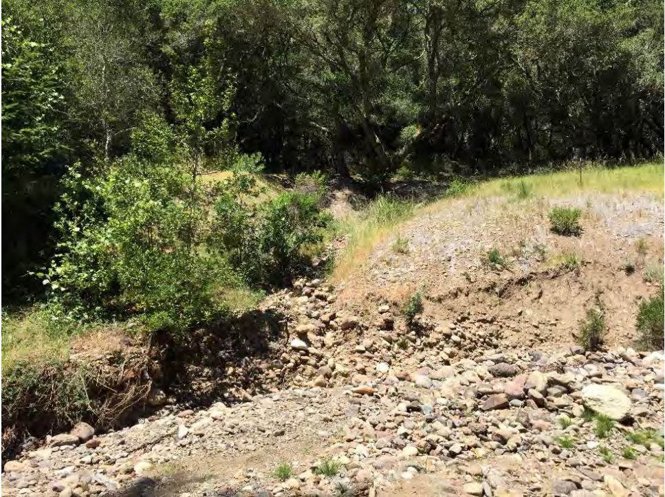
PWA Site # 25 (May 2015)
