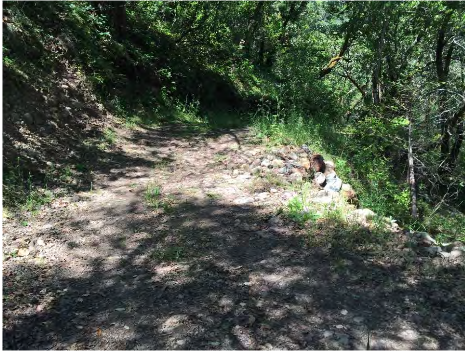
PWA Site # 20 (May 2015)
