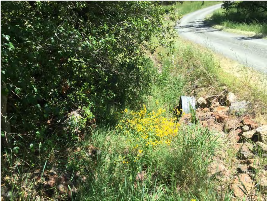
PWA Site #2 (May 2016)
