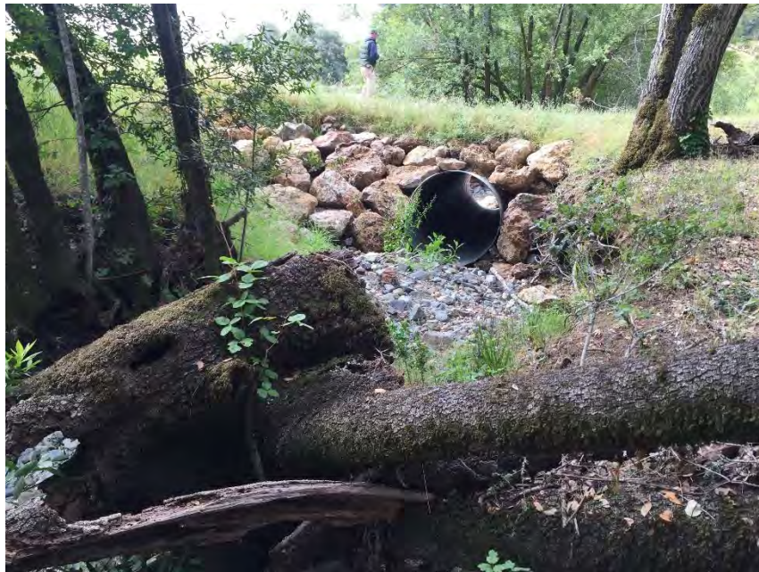
PWA Site #6 inlet (May 2015)
