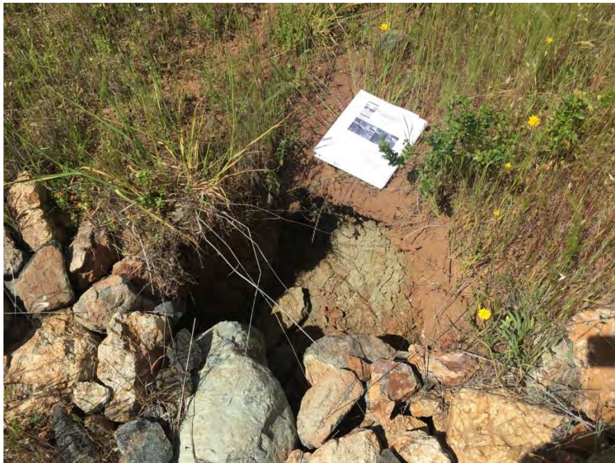
PWA Site #8.1 Grade Control Structure Headcut (May 2016)
