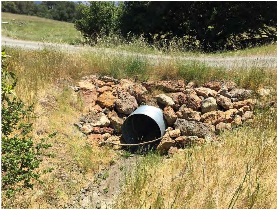
PWA Site #5 inlet (May 2015)
