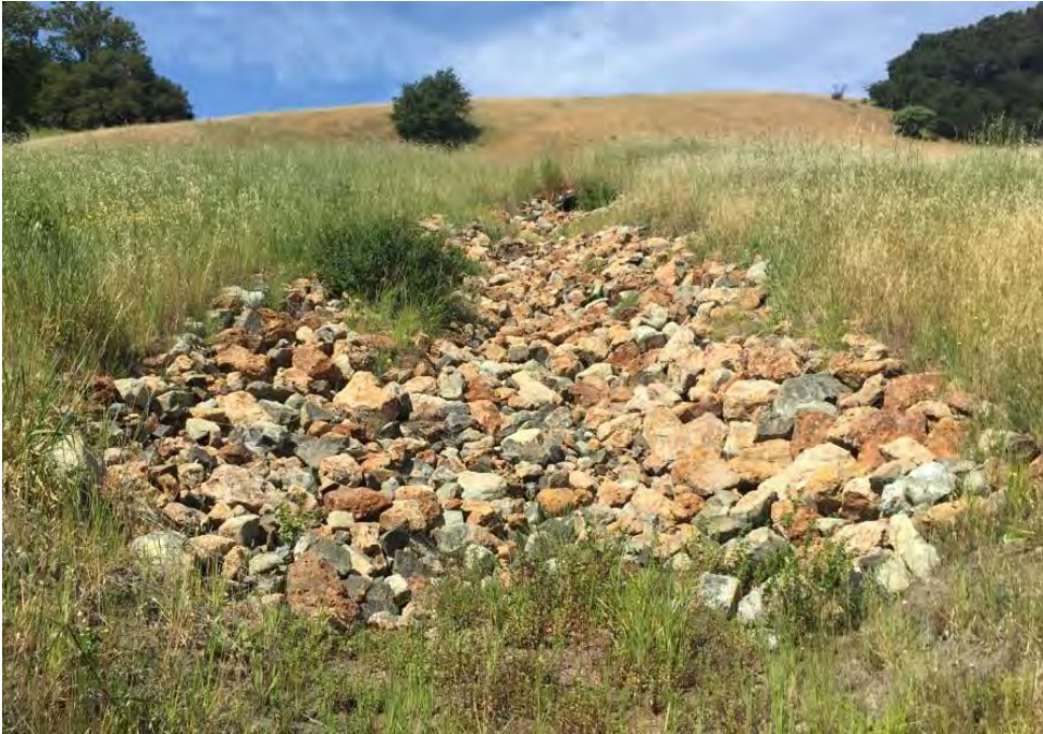
PWA Site # 8.1 (May 2016)
