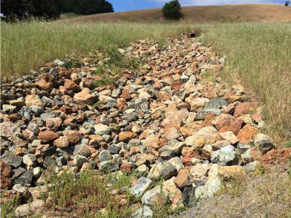
PWA Site #8.1 (May 2015)
