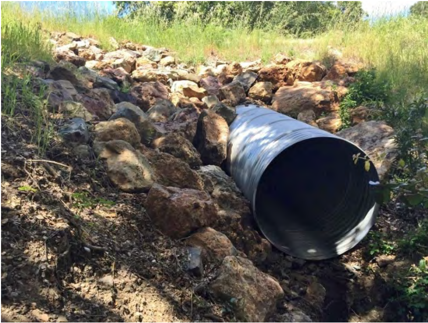
PWA Site #5 outlet (May 2016)
