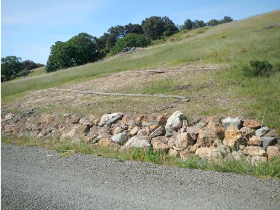
PWA Site 7.2 (May 2015)
