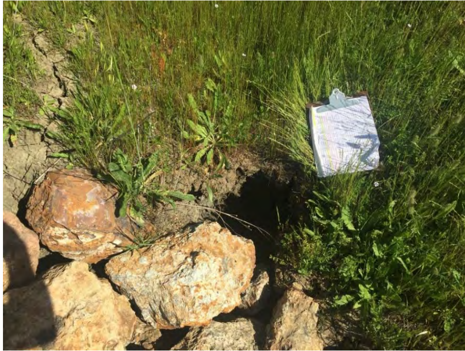
PWA Site 7.2a - Hole where inboard road ditch drains to rock armor (May 2016)
