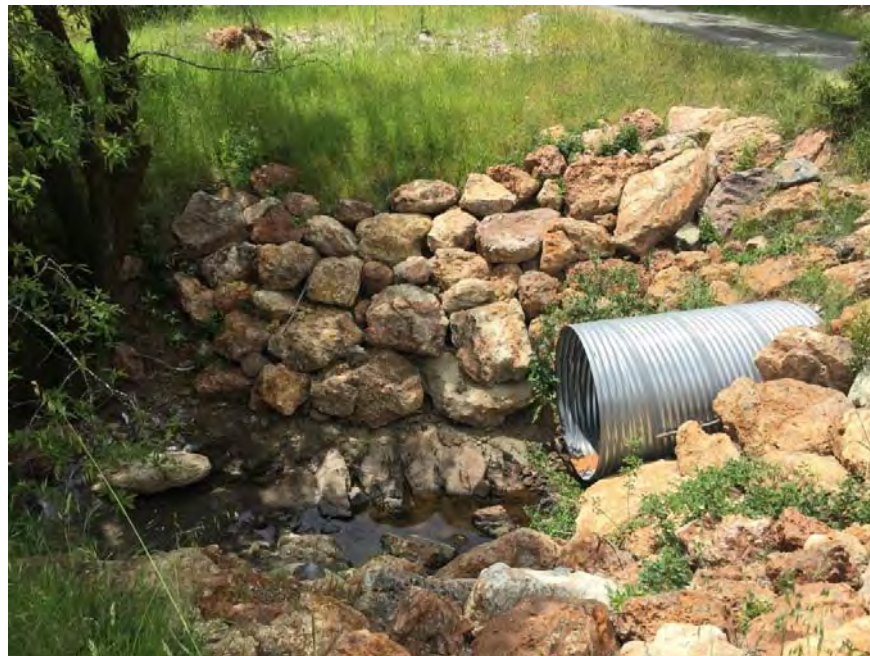
PWA Site #6 outlet (May 2016). Repair work on 9/26/2015.
