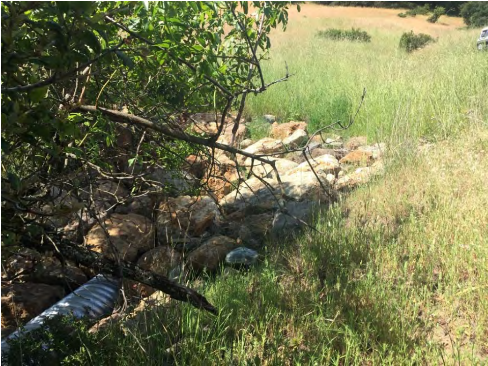
PWA Site #7 (May 2016)
