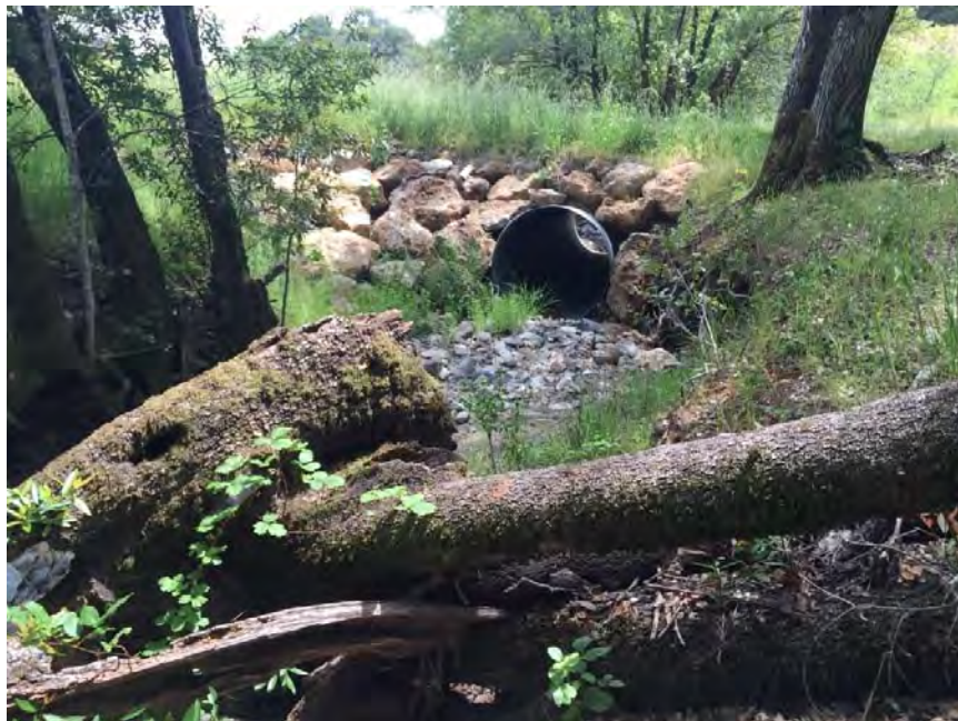
PWA Site #6 inlet (May 2016)
