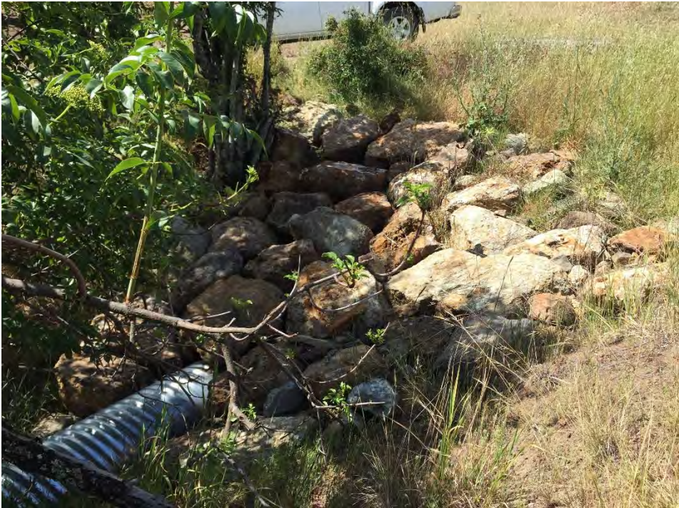
PWA Site #7 (May 2015)
