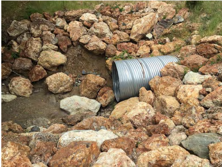
PWA Site #6 outlet (May 2015)
