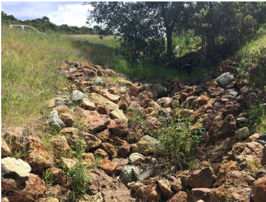
PWA Site #11 (May 2016)
