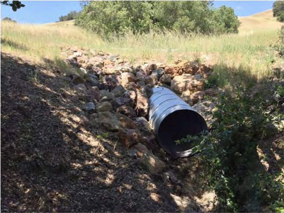
PWA Site #5 outlet (May 2015)
