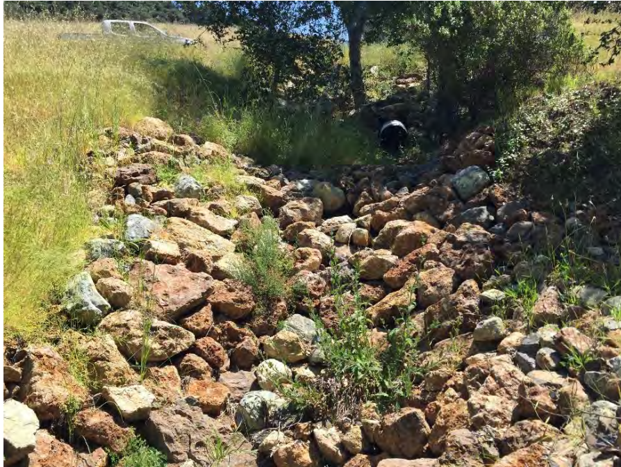
PWA Site # 11 (May 2015)
