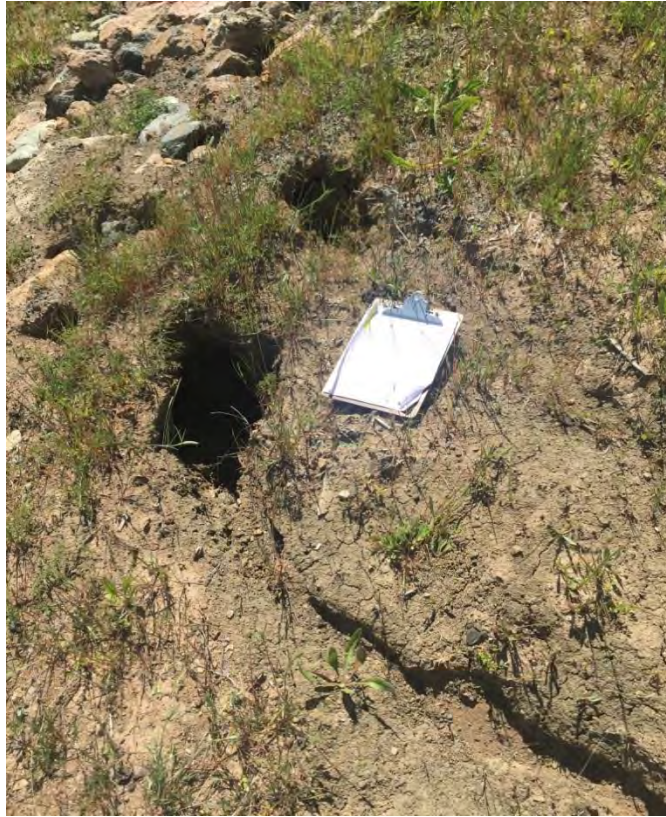
PWA Site 7.2c Rill into hole above rock armor one of two sets (May 2016)
