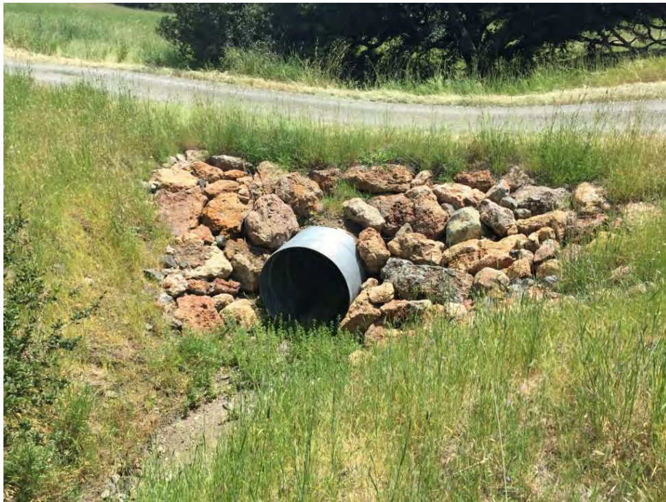
PWA Site #5 inlet (May 2016)
