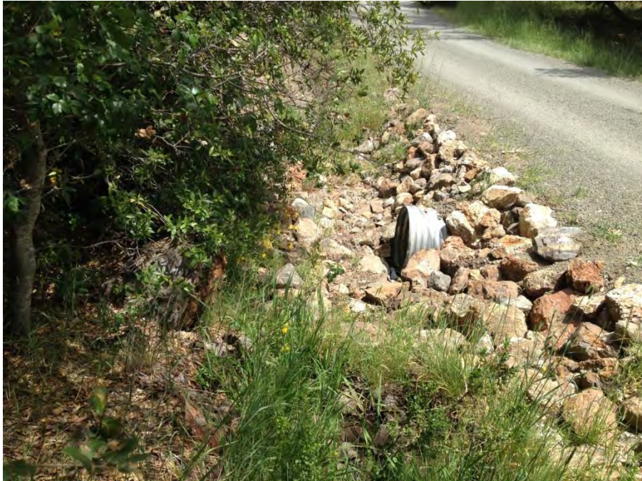
PWA Site #2 (May 2015)
