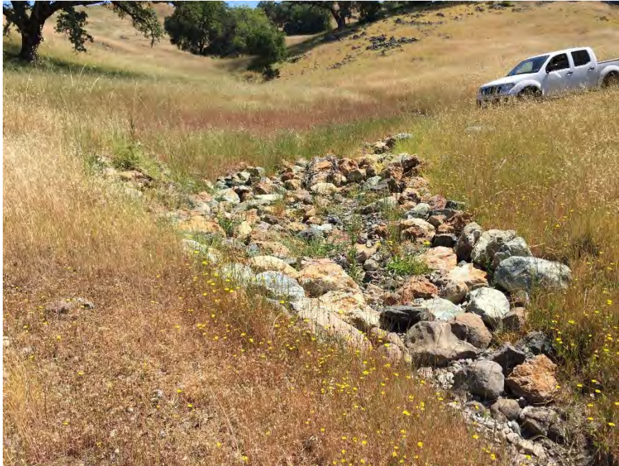
PWA Site #33 uphill (May 2015)
