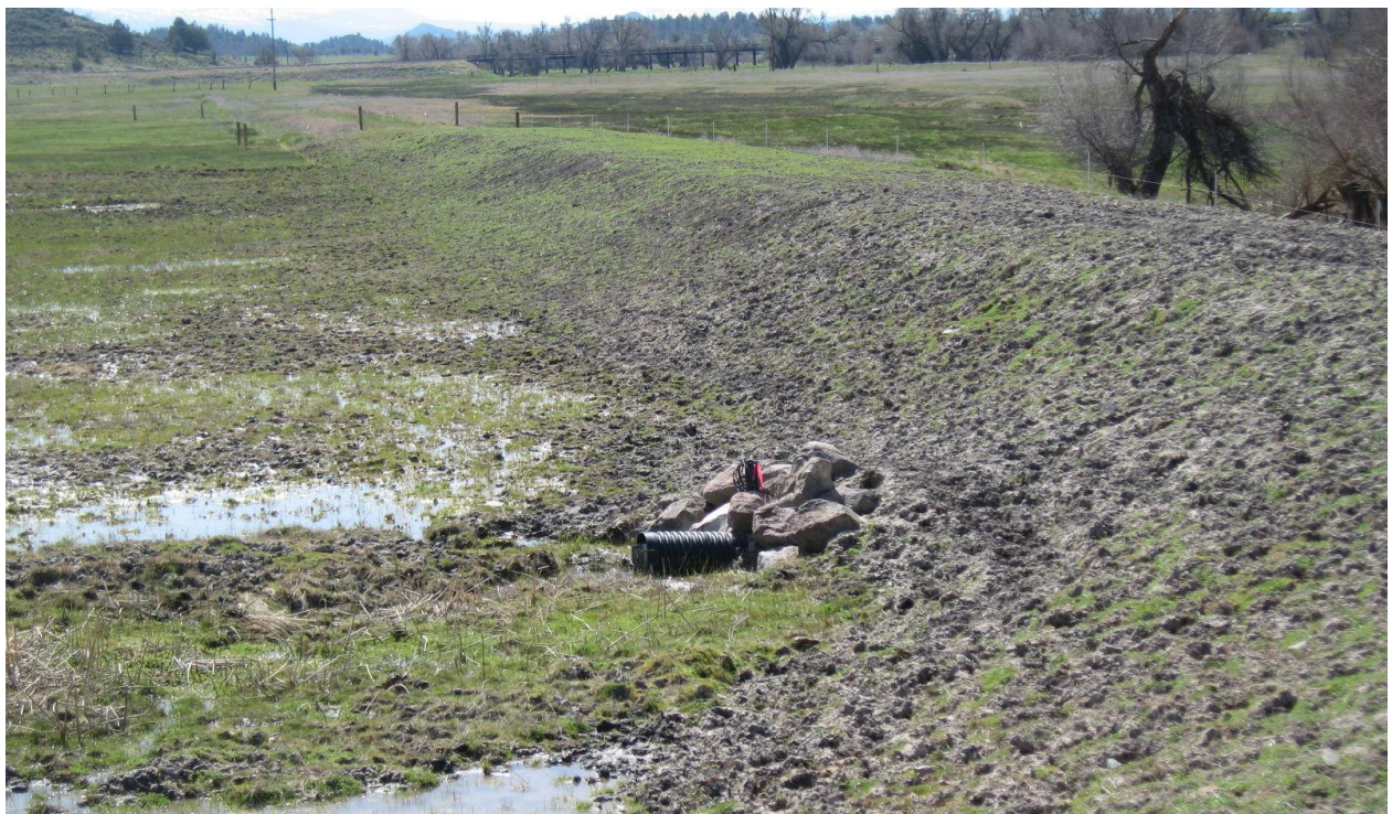
Photo: Site 03-192TW Tailwater accumulated in this low-lying area and flowed through the black culvert (in the center of the photo) to be returned to the Shasta River
