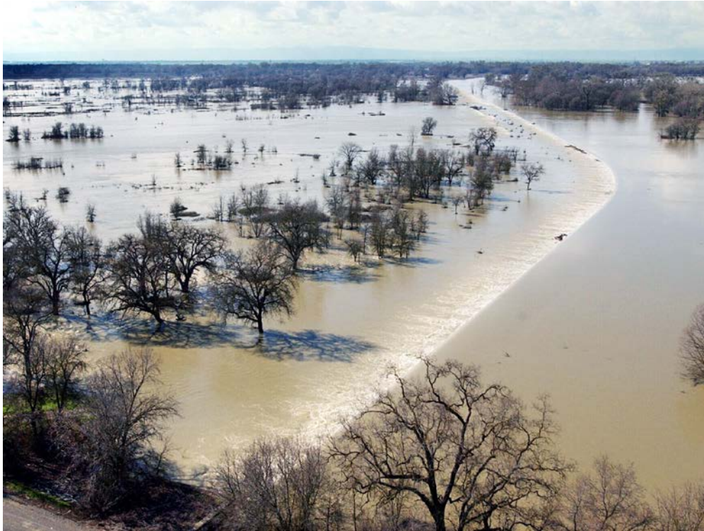
Figure 6.2-4. Example photograph of the flooding of the Yolo Bypass at the Fremont Weir. SOURCE: Randy Pench/The Sacramento Bee/Zuma Press.
